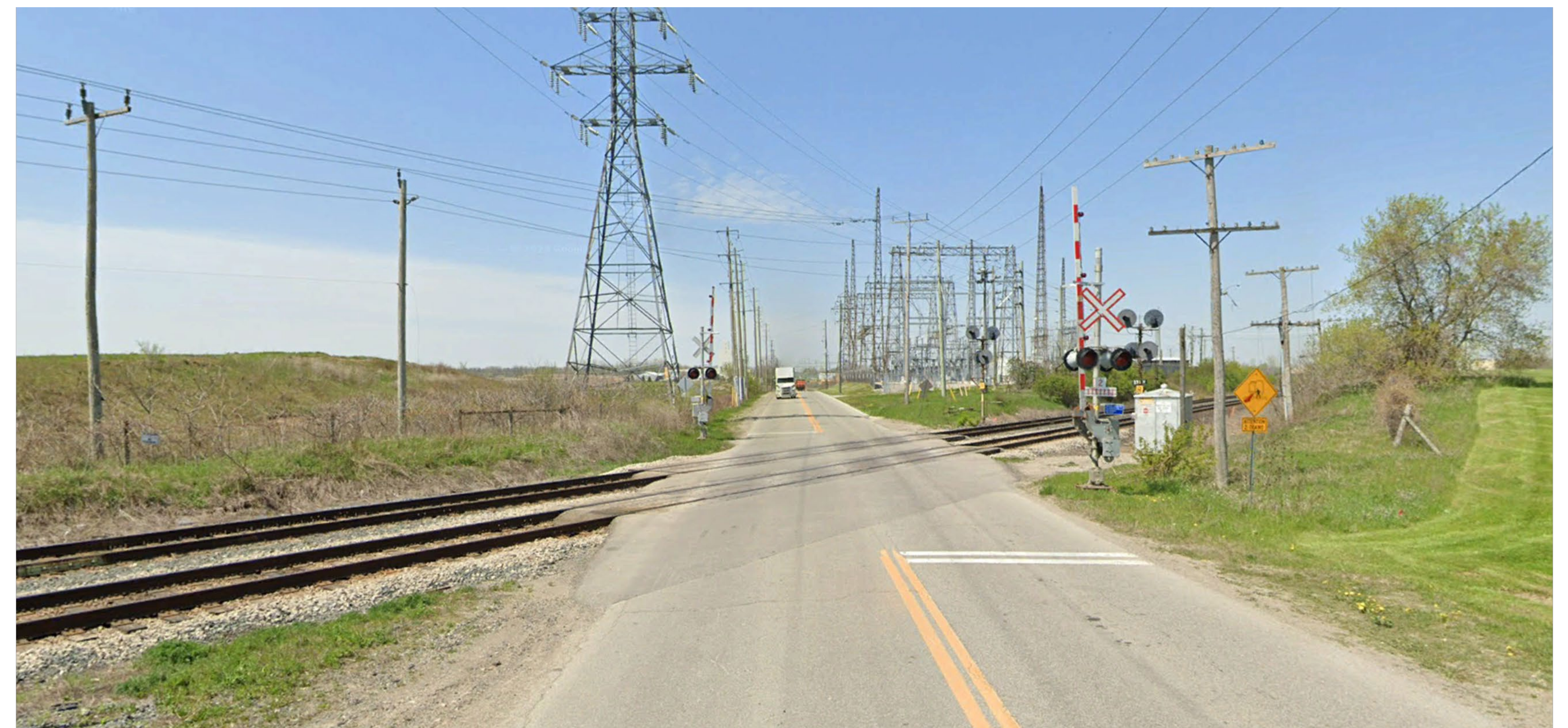
Powerline Road west of Paris Road, looking west
