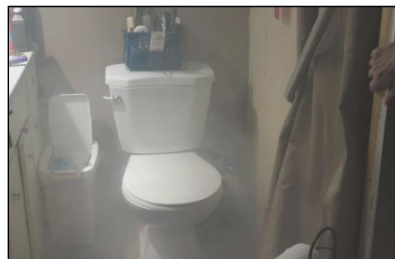
Smoke out of plumbing vent and internal plumbing indicating a connection with storm sewer.
