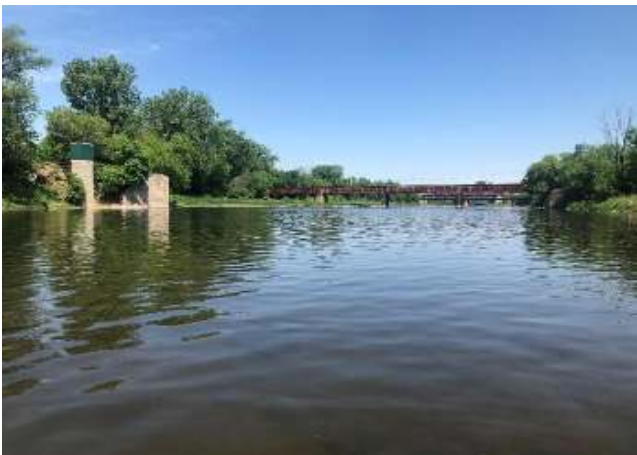
Photograph 7: Facing upstream 200 m downstream from TH&B Rail Bridge.
