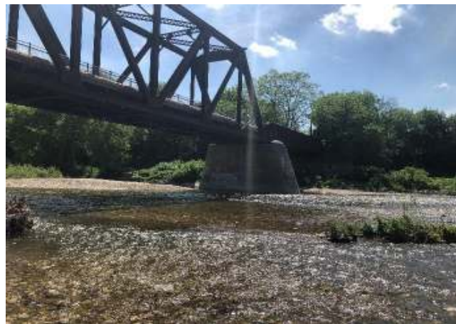
Photograph 4: Facing right downstream bank on upstream side of Brant's crossing Bridge.
