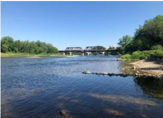
Photograph 7: Facing upstream 200 m downstream of Brant's Crossing Bridge.
