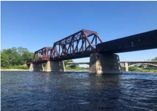
Photograph 5: Downstream side of Brant's Crossing Bridge facing towards right downstream bank.
