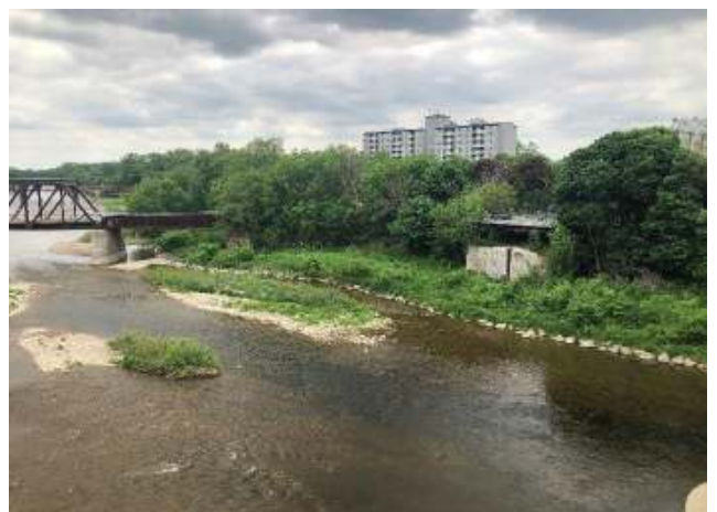
Photograph 10: Facing right downstream bank from Lorne Bridge.
