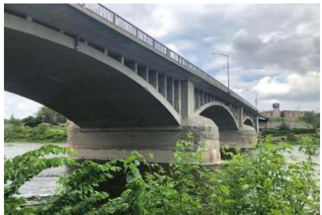
Photograph 10: Downstream side of Lorne Bridge.
