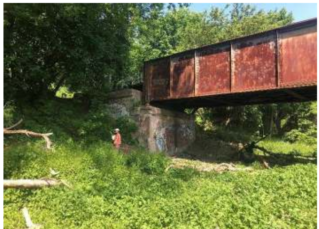
Photograph 10: Facing downstream side of west bridge abutment - TH&B Rail Bridge.
