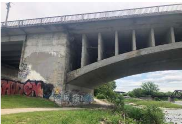
Photograph 9: Upstream side of east Lorne bridge abutment.
