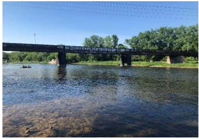
Photograph 8: Facing downstream 200 m downstream of Brant's Crossing Bridge.
