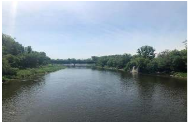
Photograph 2: Facing downstream from TH&B Rail Bridge.
