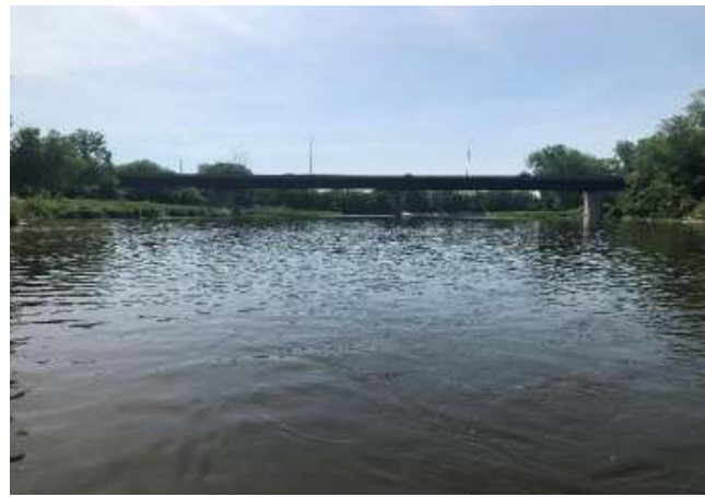
Photograph 8: Facing downstream 200 m downstream from TH&B Rail Bridge.
