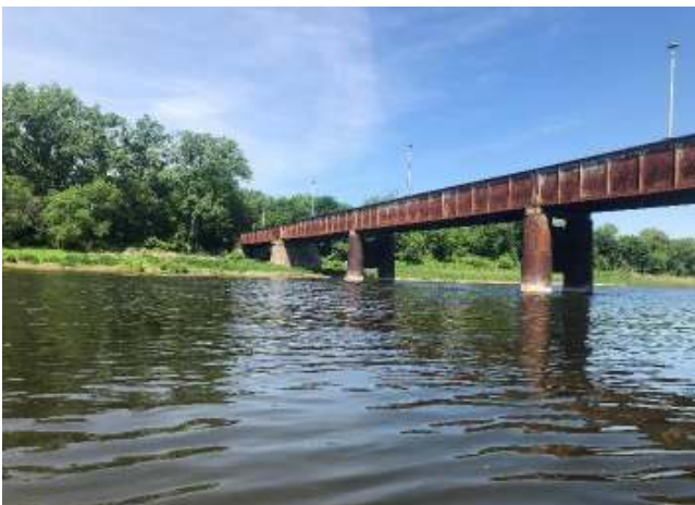
Photograph 9: Facing downstream side of TH&B Rail Bridge from left downstream bank.
