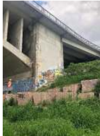
Photograph 8: Downstream side of east Lorne bridge abutment.
