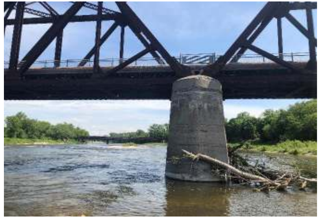
Photograph 6: Facing downstream 200m D/S from Lorne Bridge.
