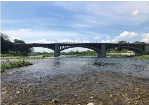
Photograph 5: Facing upstream 200m D/S from Lorne Bridge.
