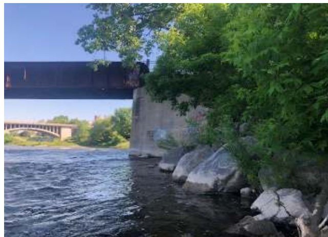
Photograph 10: Downstream side of east bridge abutment of Brant's Crossing Bridge.
