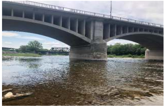
Photograph 2: Facing downstream 50 m upstream from Lorne Bridge.
