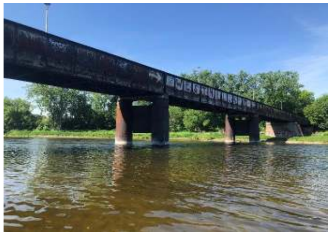
Photograph 4: Facing upstream side of TH&B Rail Bridge from east bank.
