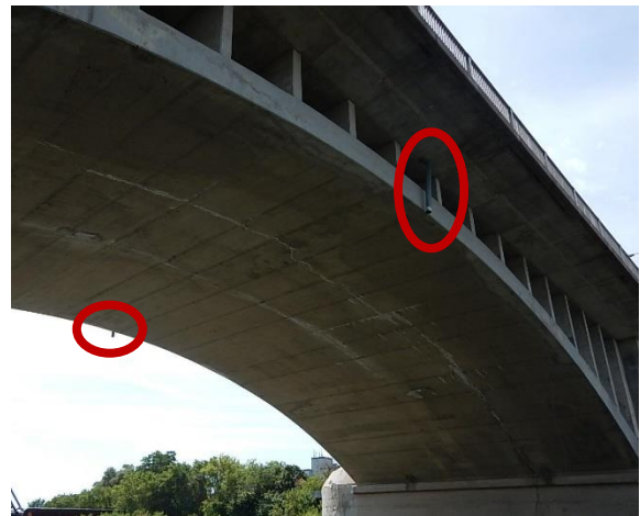
Figure 2: Deck deck drain outlets at center arch
