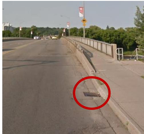
Figure 4: North catch basin at east end of Lorne Bridge
