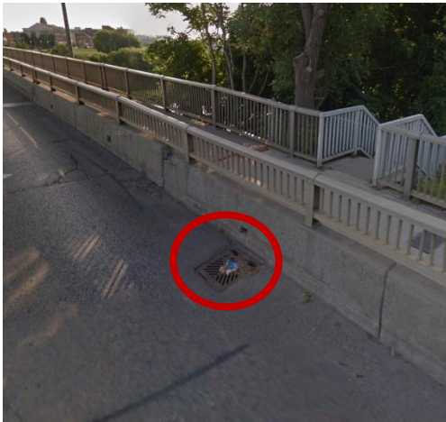
Figure 3: South catch basin at west end of Lorne Bridge
