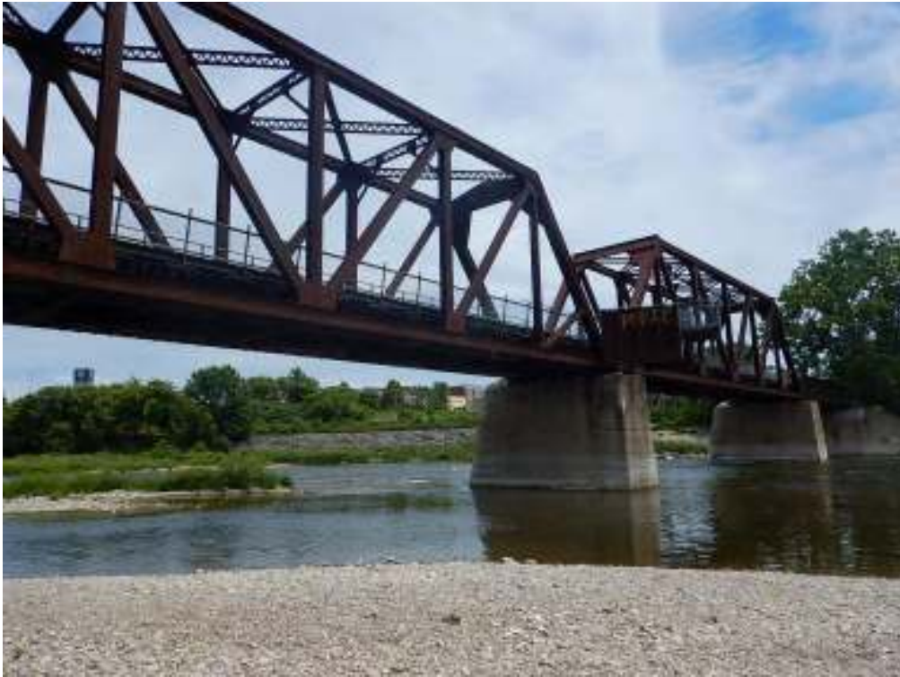
Photograph T1: Truss bridge span, south elevation
