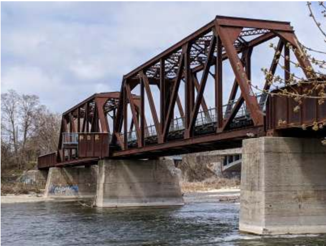
Figure 39: Downriver sides of the piers, facing northwest
