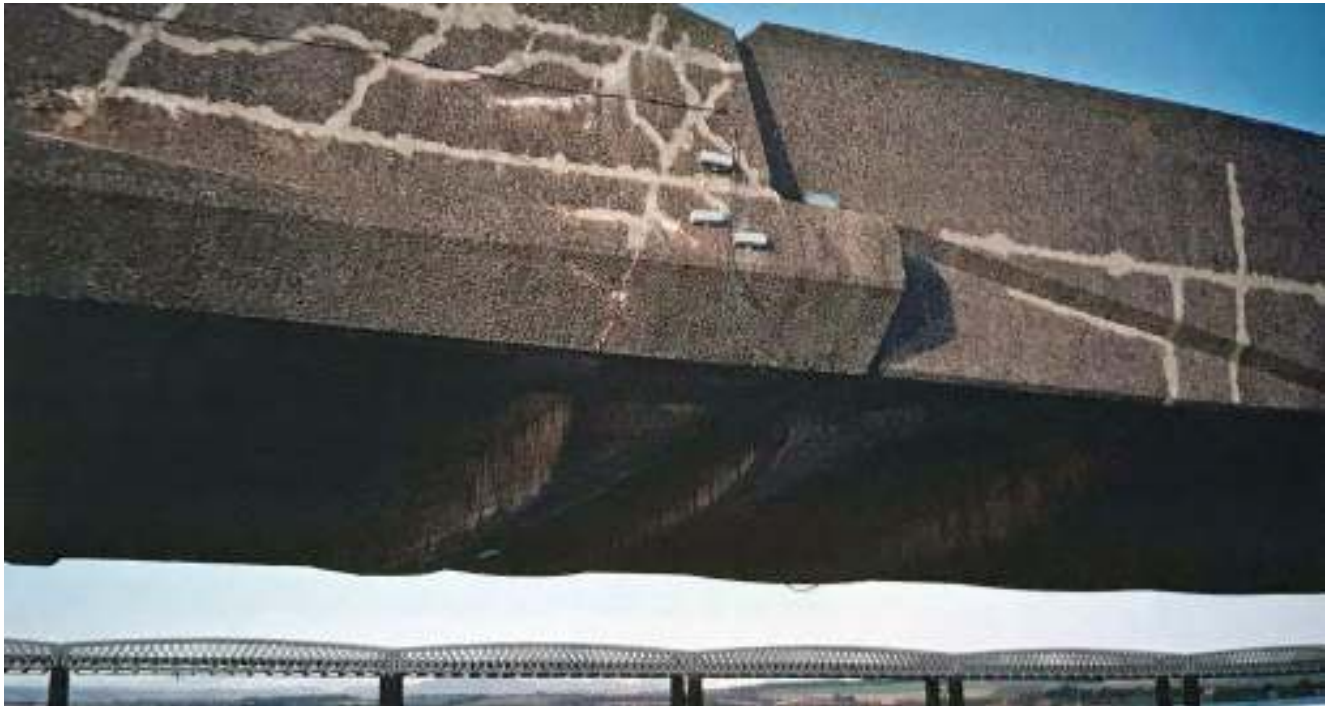
Figure 78: Example of an inappropriate crack repair, Montrose Bridge, Scotland (English Heritage 2018:182)
