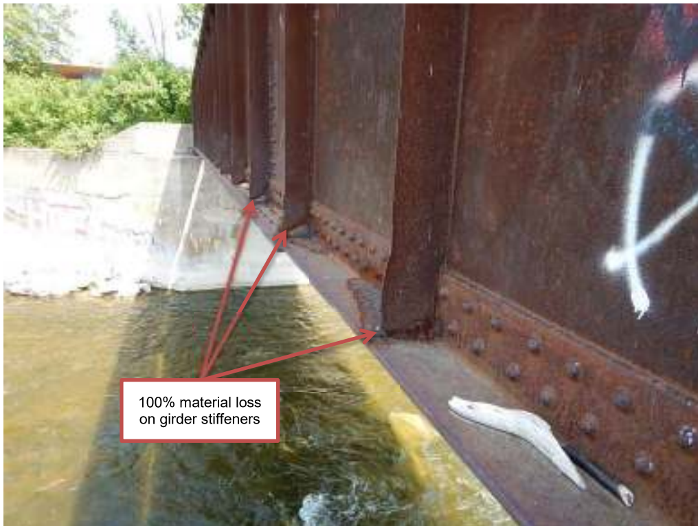
Photograph G10: East span, north girder exterior
