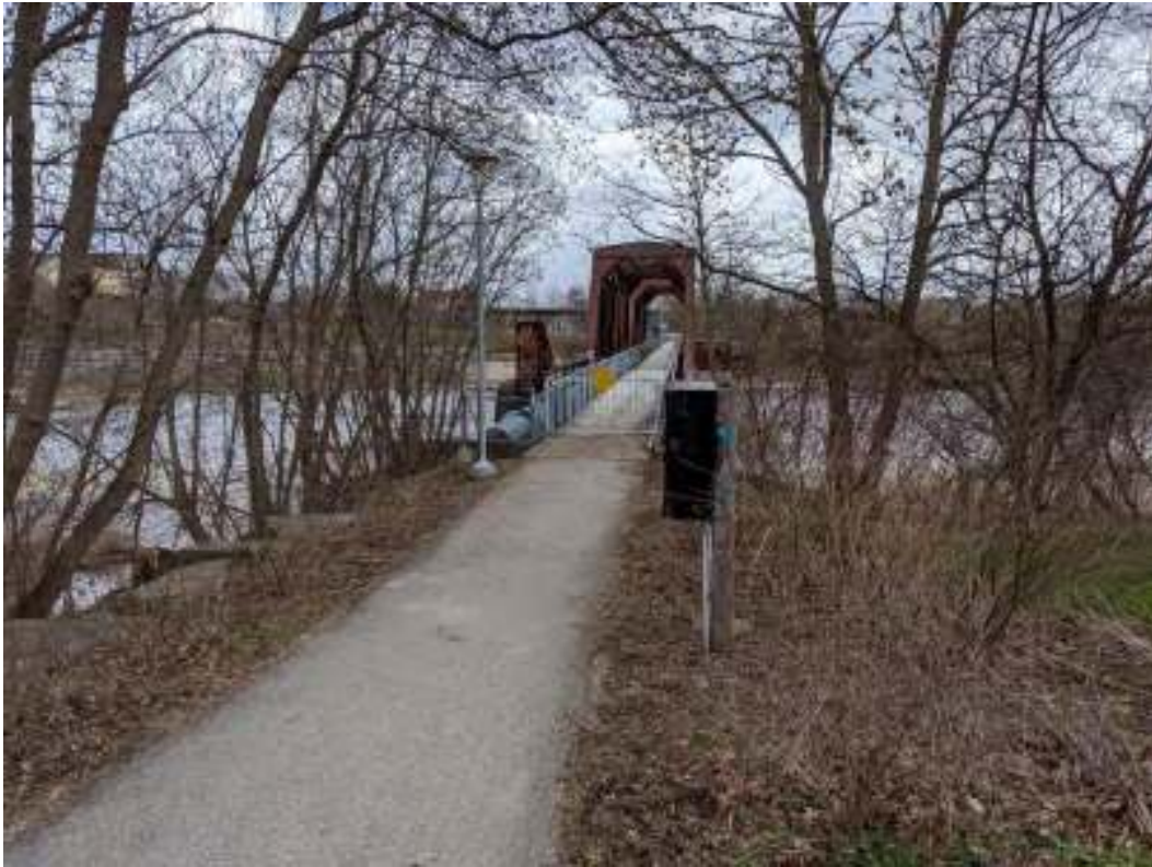
Figure 31: West approach to Brant's Crossing
