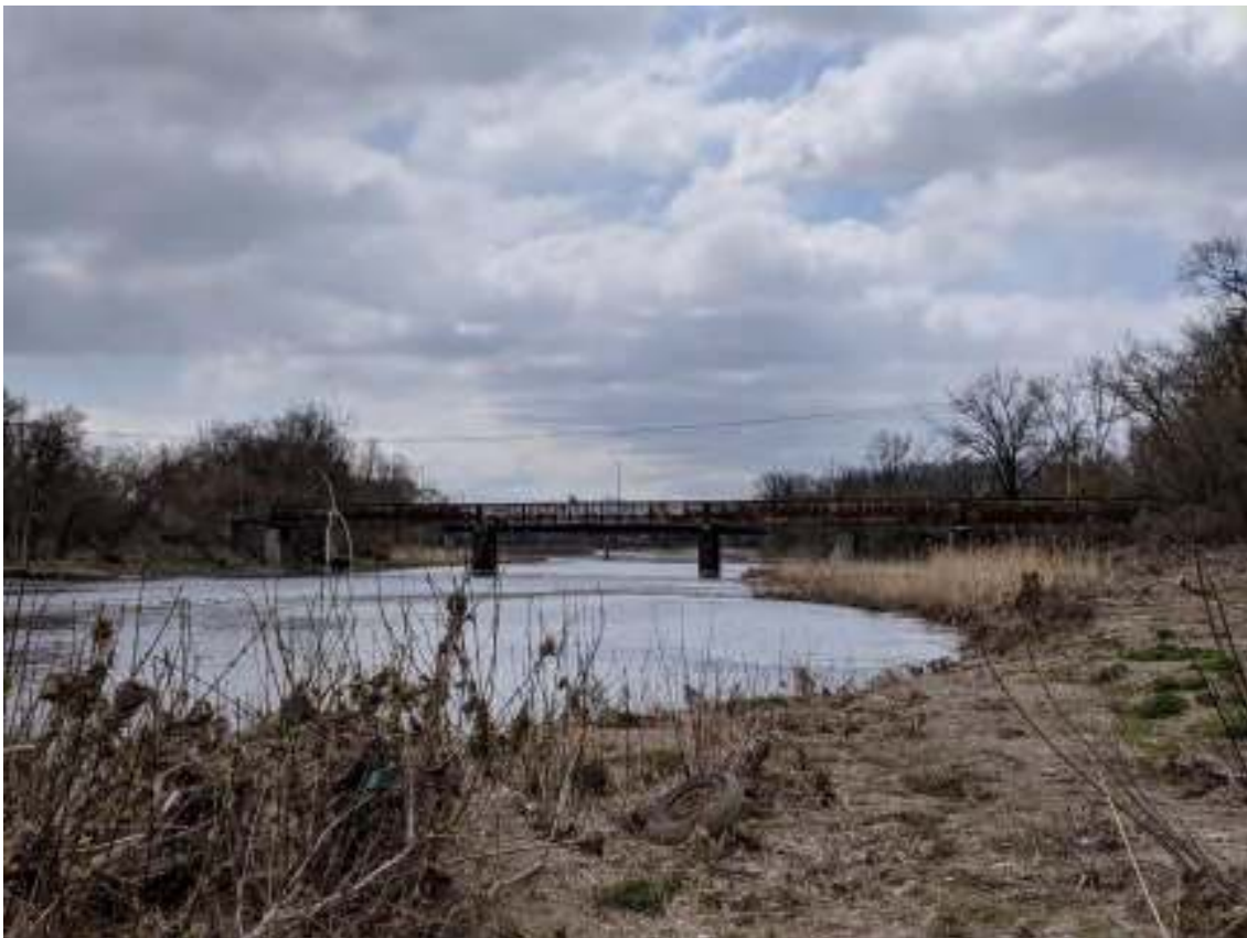
Figure 54: Setting of the TH&B Crossing Bridge, facing south from the west bank below Brant's Crossing Bridge
