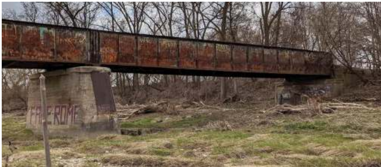
Figure 62: View facing southwest of the west abutment and pier
