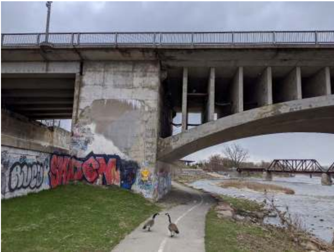
Figure 15: North side of the east abutment of the Lorne Bridge
