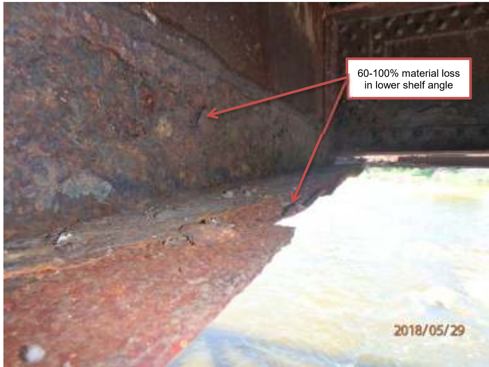
Photograph T11: East truss (Floor beam #10)
