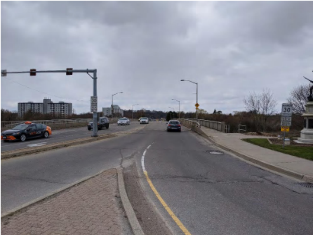
Figure 5: View facing west of the east approach
