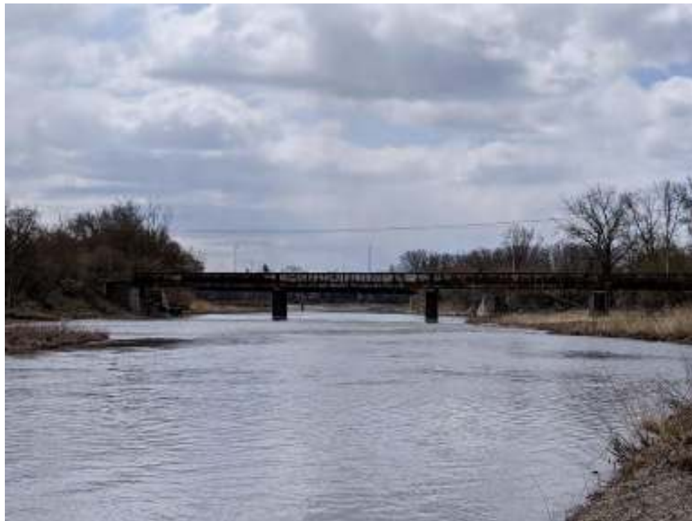
Figure 34: View downriver of the TH&B Crossing Bridge
