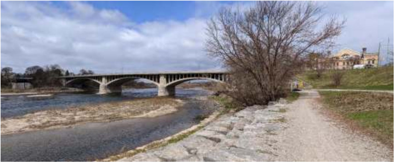
Figure 3: View of the Lorne Bridge facing north from the east bank
