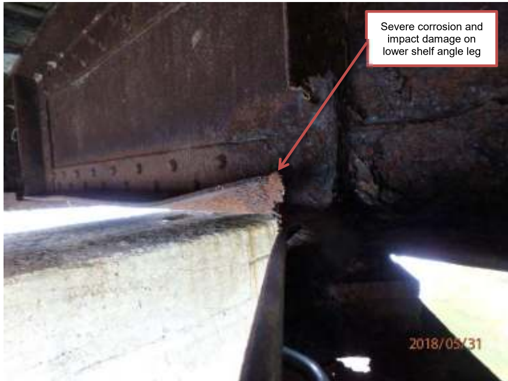
Photograph G12: West span, north stringer
