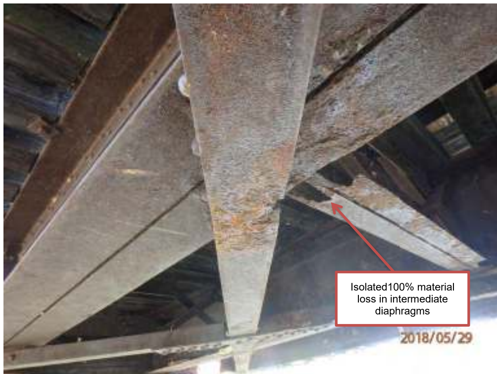
Photograph T12: East truss, underside
