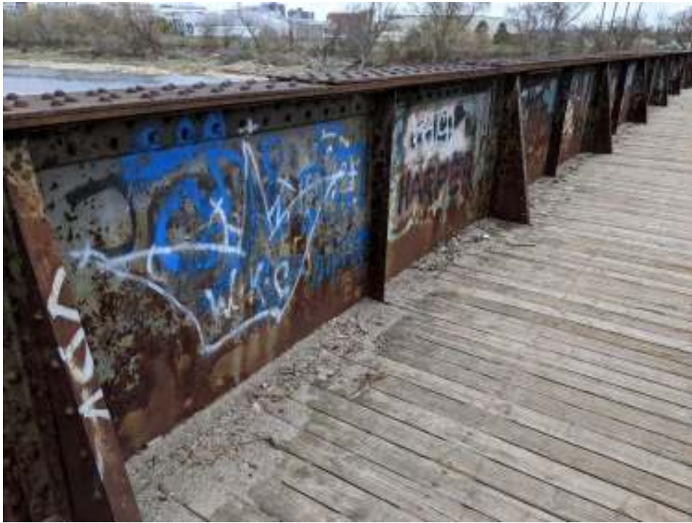
Figure 73: Interior side of the girders, showing the top flange plate and rectangular and triangular vertical web stiffeners
