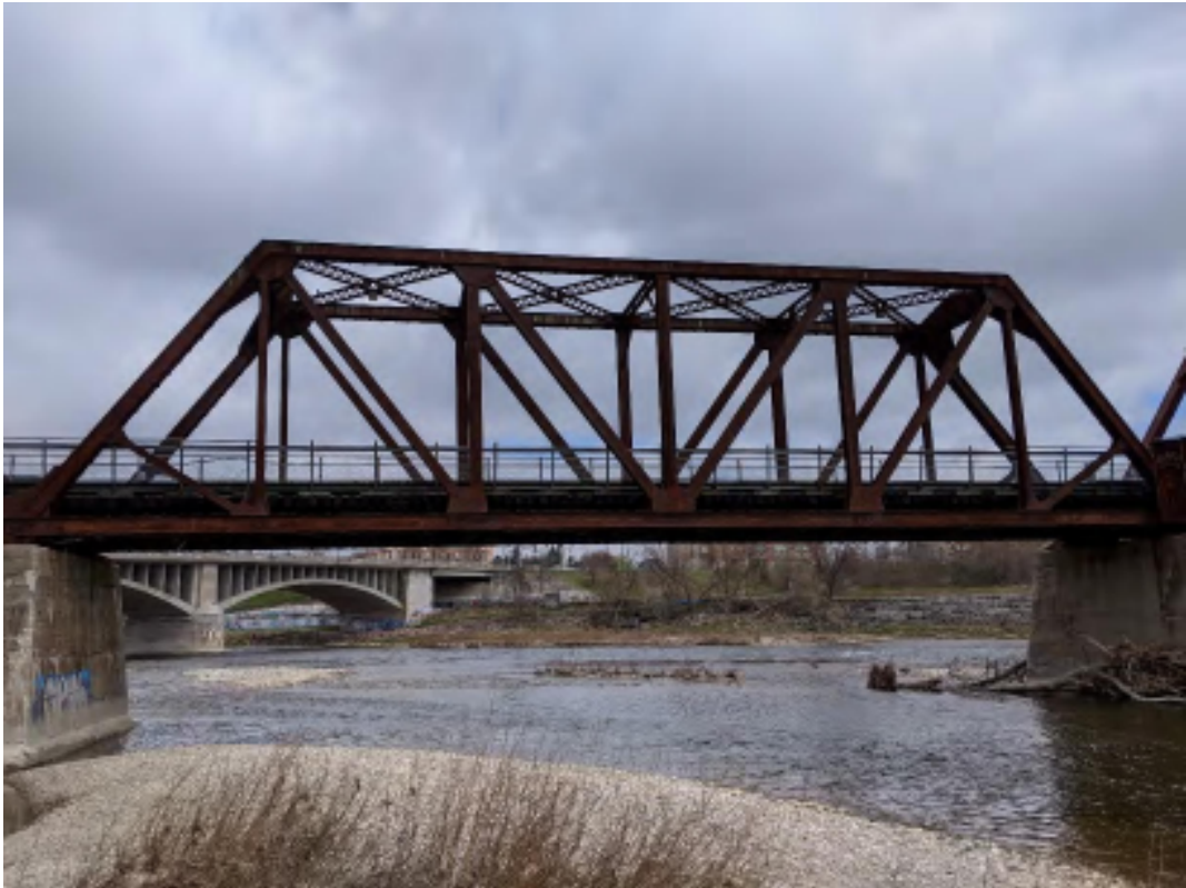
Figure 46: South side of the west Pratt through truss span
