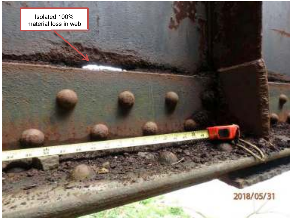
Photograph G7: West span, north girder
