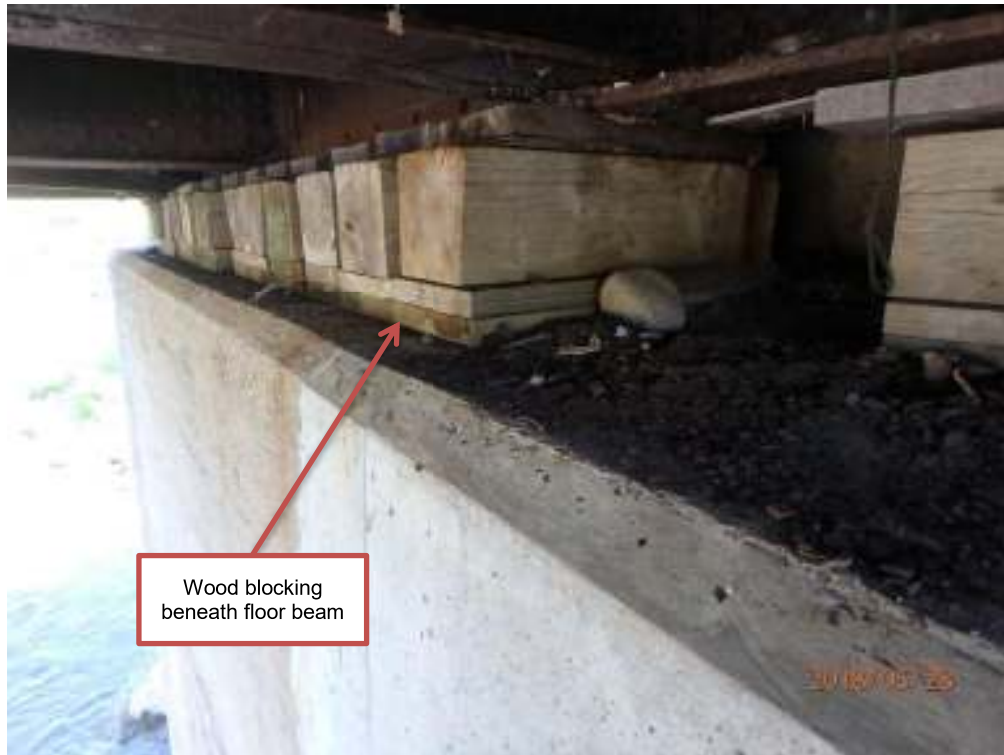
Photograph G3: East abutment
