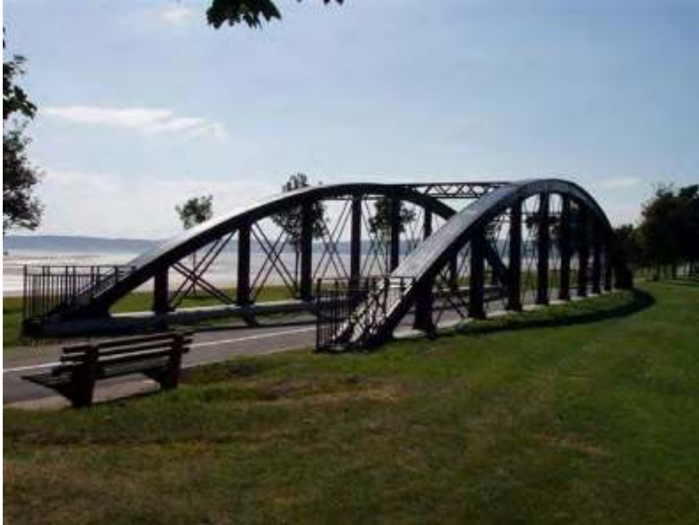
Figure 81: Example of a relocated truss bridge. The Swansea Slip Bridge in Swansea, Wales dates to 1914 and was relocated intact to a public park in 2004 (Dalling 2018)
