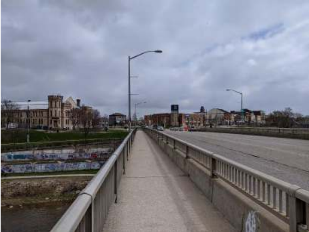
Figure 6: View east from the Lorne Bridge
