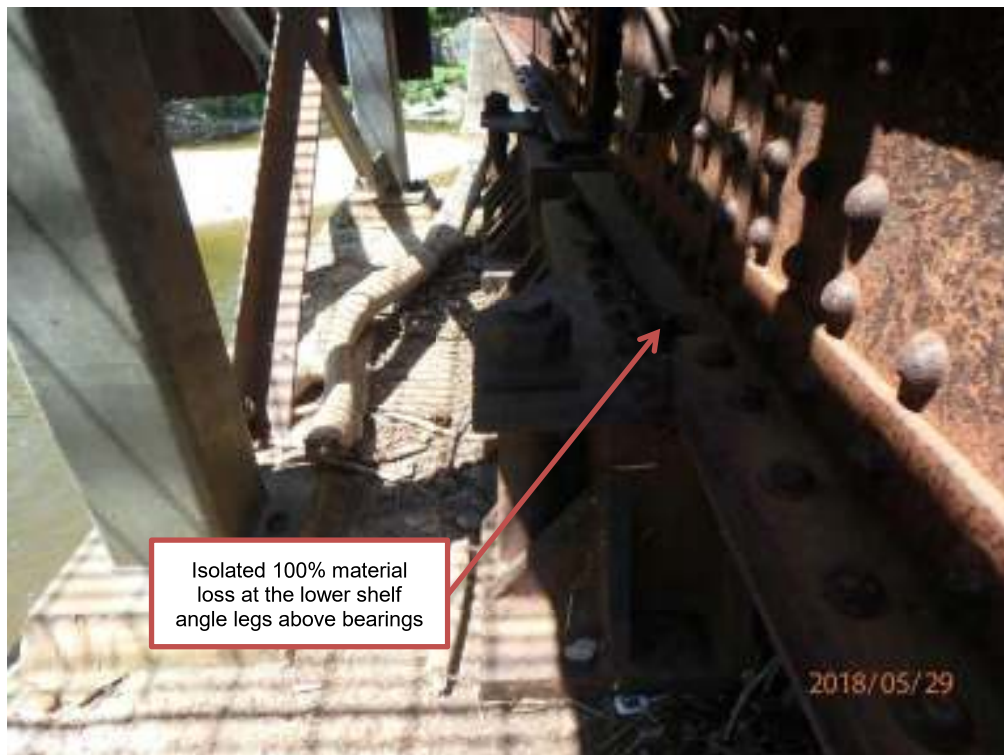
Photograph T6: Centre pier, southeast bearing
