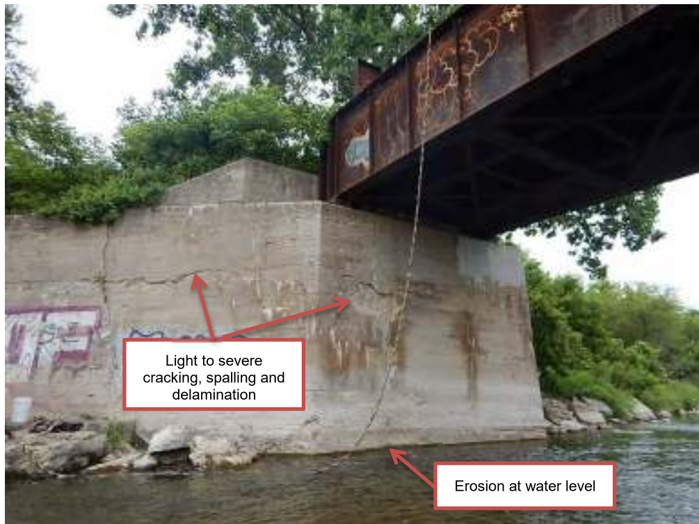
Photograph G2: East Abutment
