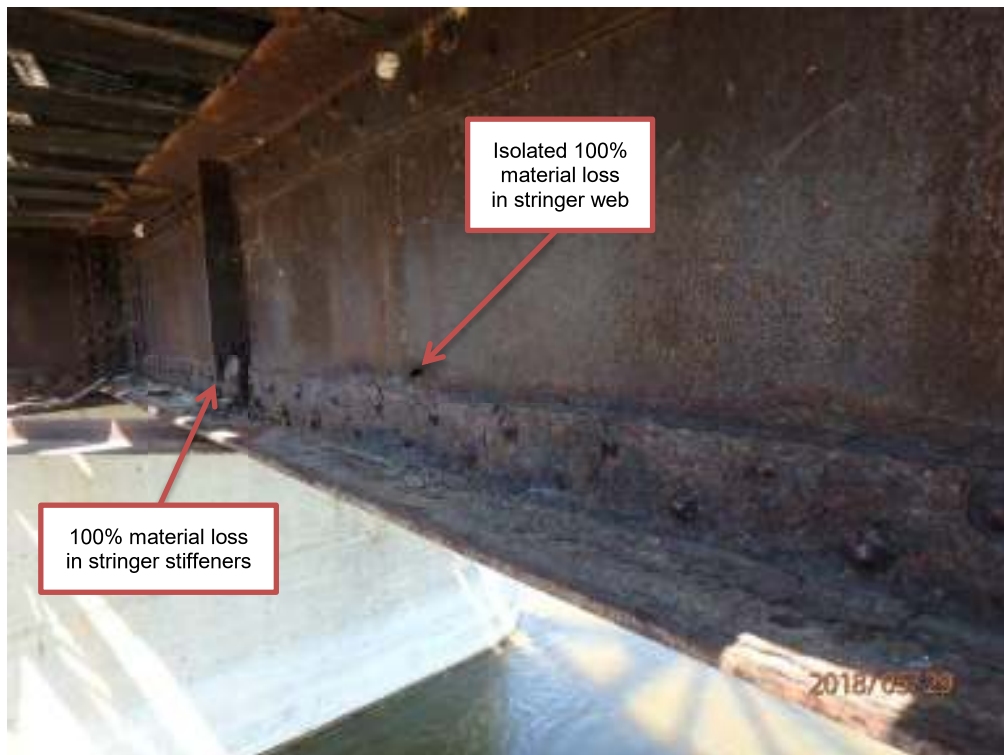
Photograph T10: East truss, south stringer
