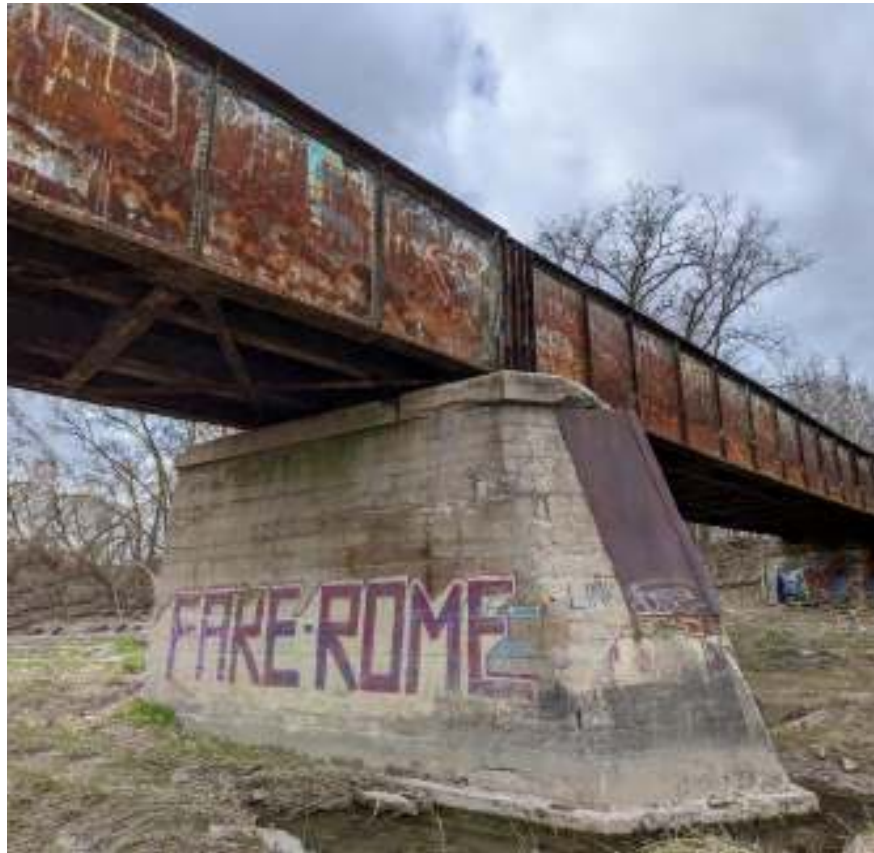
Figure 67: View facing south of the concrete pier
