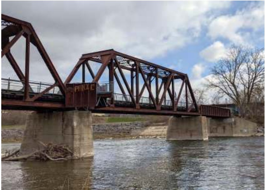
Figure 47: West and south sides of the east Pratt through truss span
