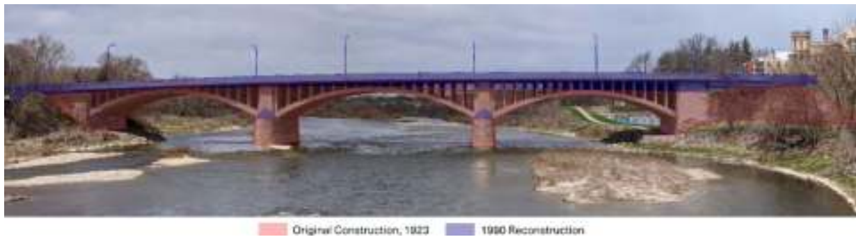
Figure 79: Comparison of the original and current Lorne Bridge configurations, with blue shading indicating where the new spandrel columns were added to the crown of the arches in 1980 (top image, the Lorne Bridge in 1924, Toronto Public Library – Toronto Star Archives)
