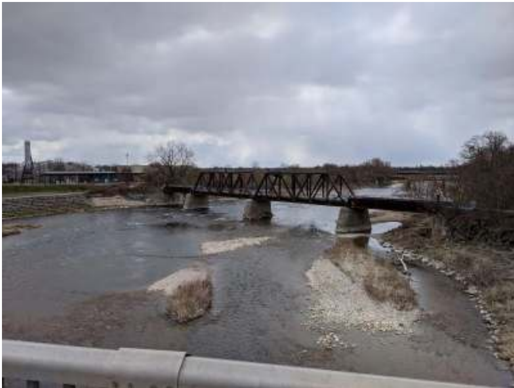
Figure 28: Setting of Brant's Crossing Bridge, facing south from the Lorne Bridge
