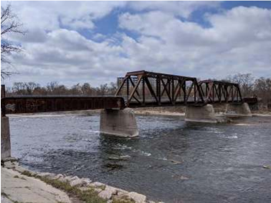
Figure 38: Upriver side of the piers, facing southwest
