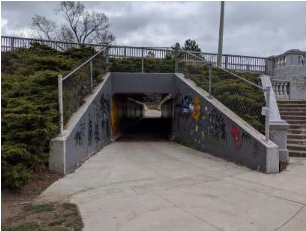
Figure 19: South headwall and wing walls of the concrete pedestrian underpass
