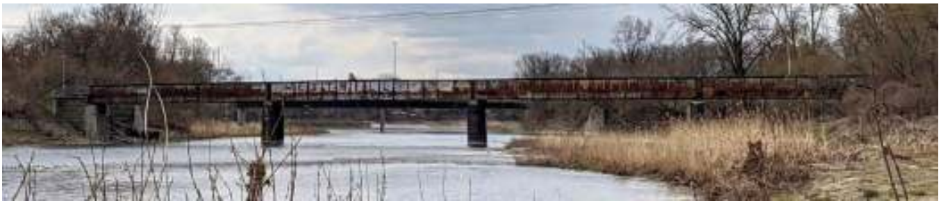
TH&B Crossing Bridge, North Elevation
