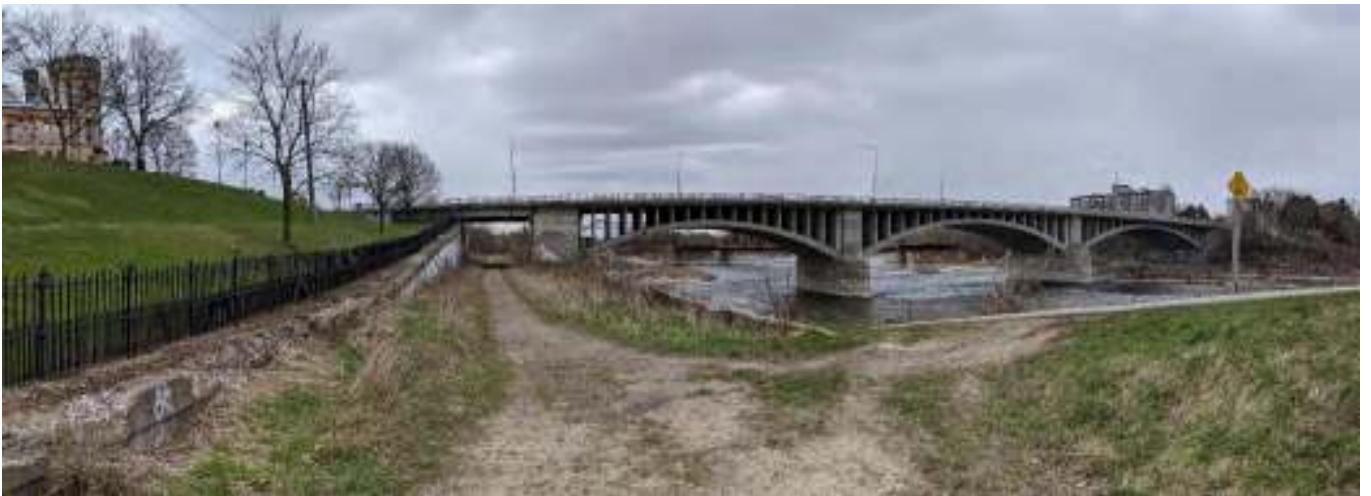
Figure 4: View of the Lorne Bridge facing south from the east bank.
