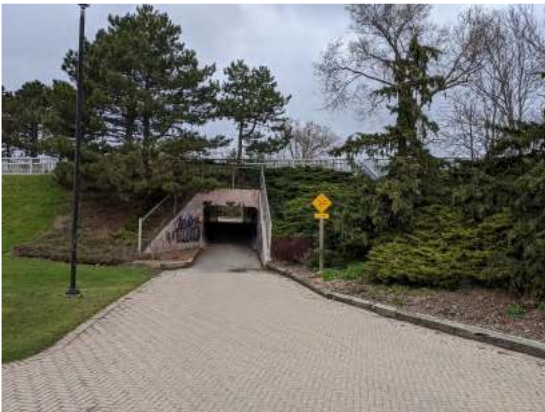
Figure 20: North headwall and wing walls of the concrete pedestrian underpass
