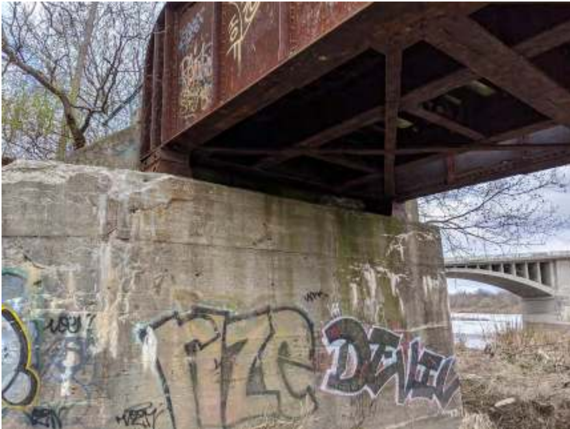
Figure 37: Front wall and ballast wall of the west abutment
