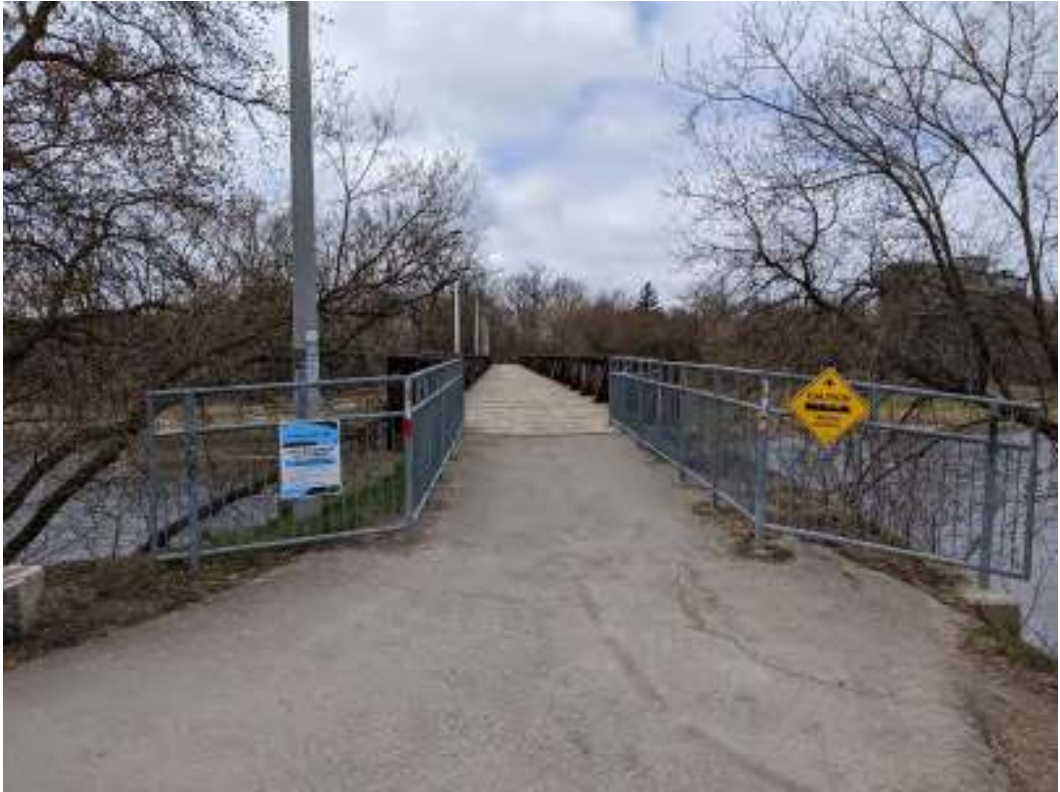
Figure 56: East approach to the TH&B Crossing Bridge, facing west
