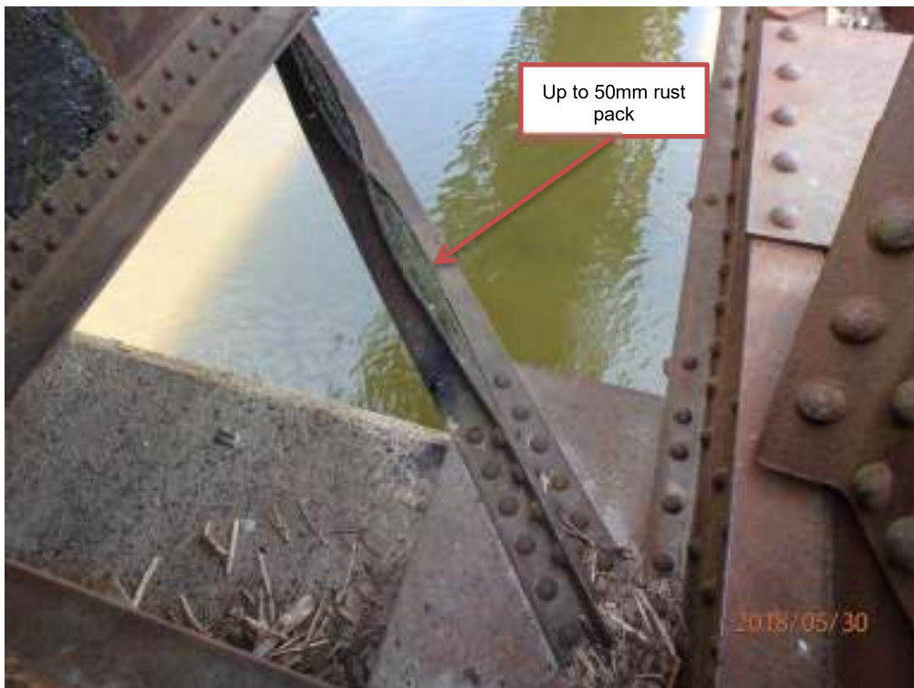
Photograph T14: West truss, lateral bracing
