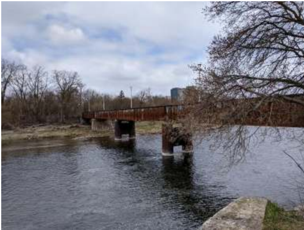
Figure 72: View facing northwest of the girder spans
