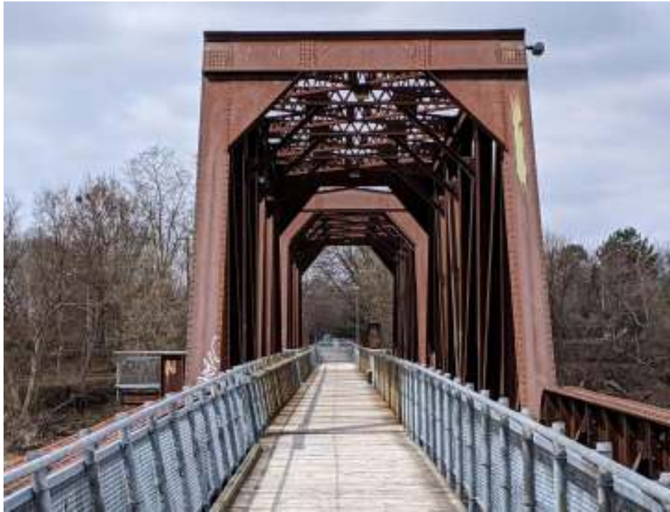
Figure 52: East portal of the east Pratt through truss span
