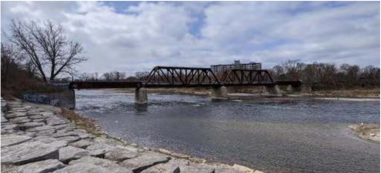
Figure 27: Setting of Brant's Crossing Bridge, facing southwest from the east bank
