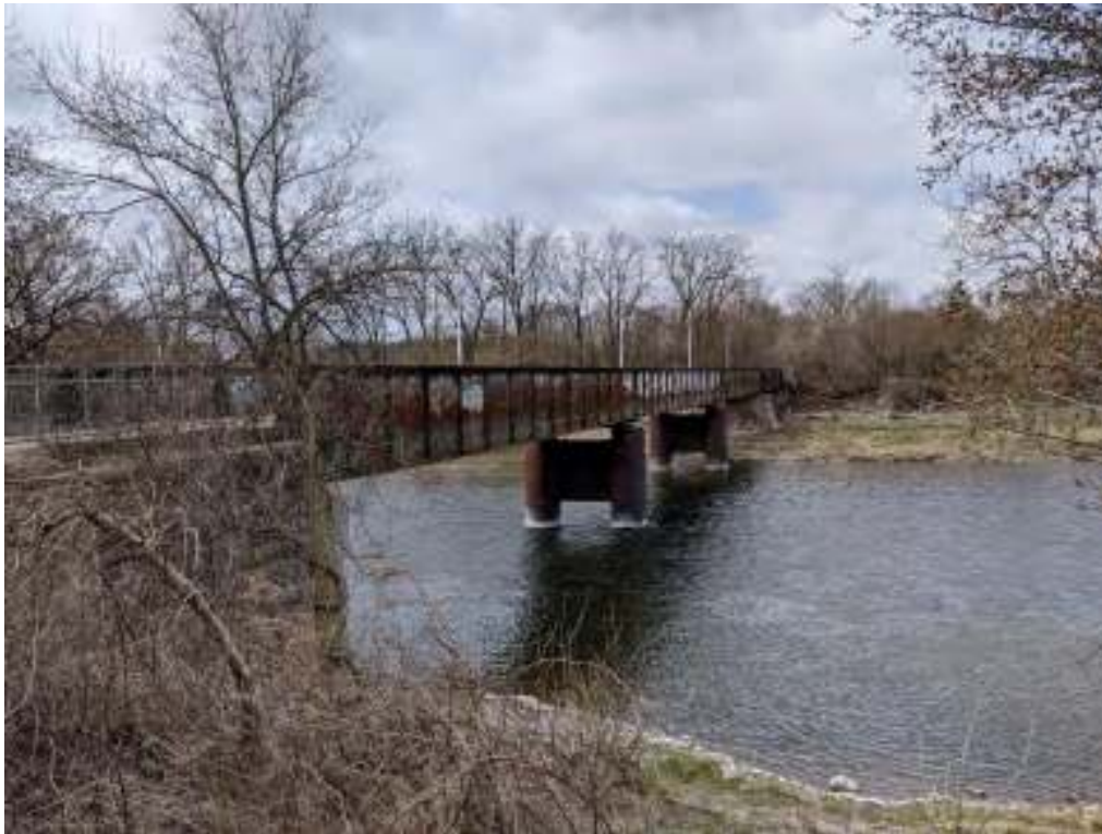
Figure 71: View facing west of the girder spans
