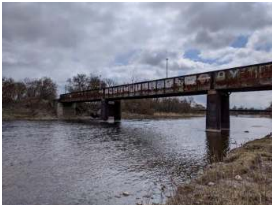
Figure 68: View facing southeast of the metal pier bents
