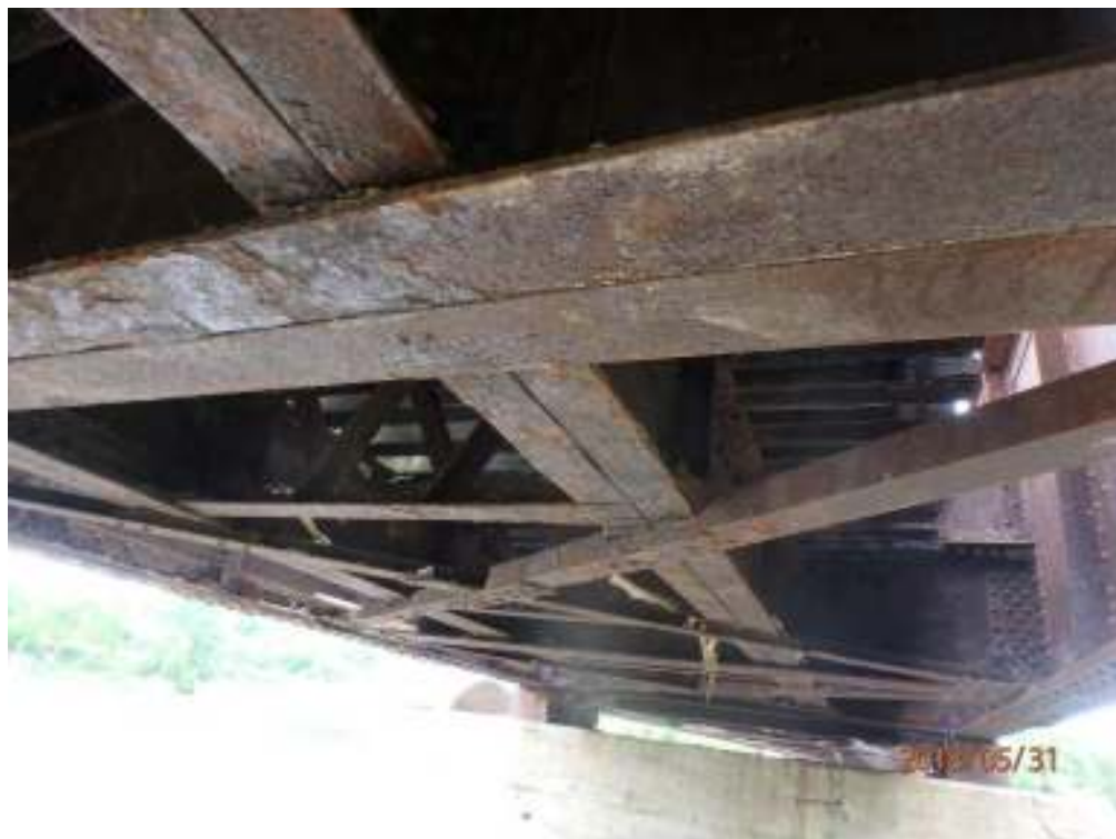
Photograph G16: West span underside
