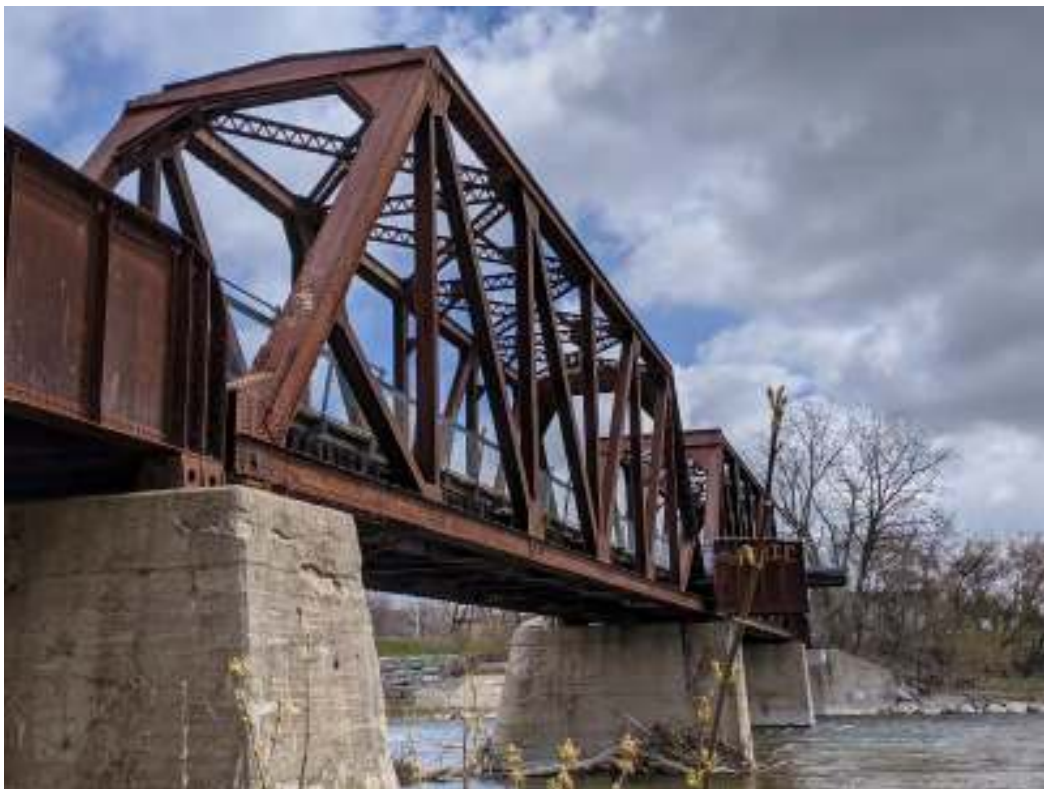
Figure 45: West and south sides of the west Pratt through truss span
