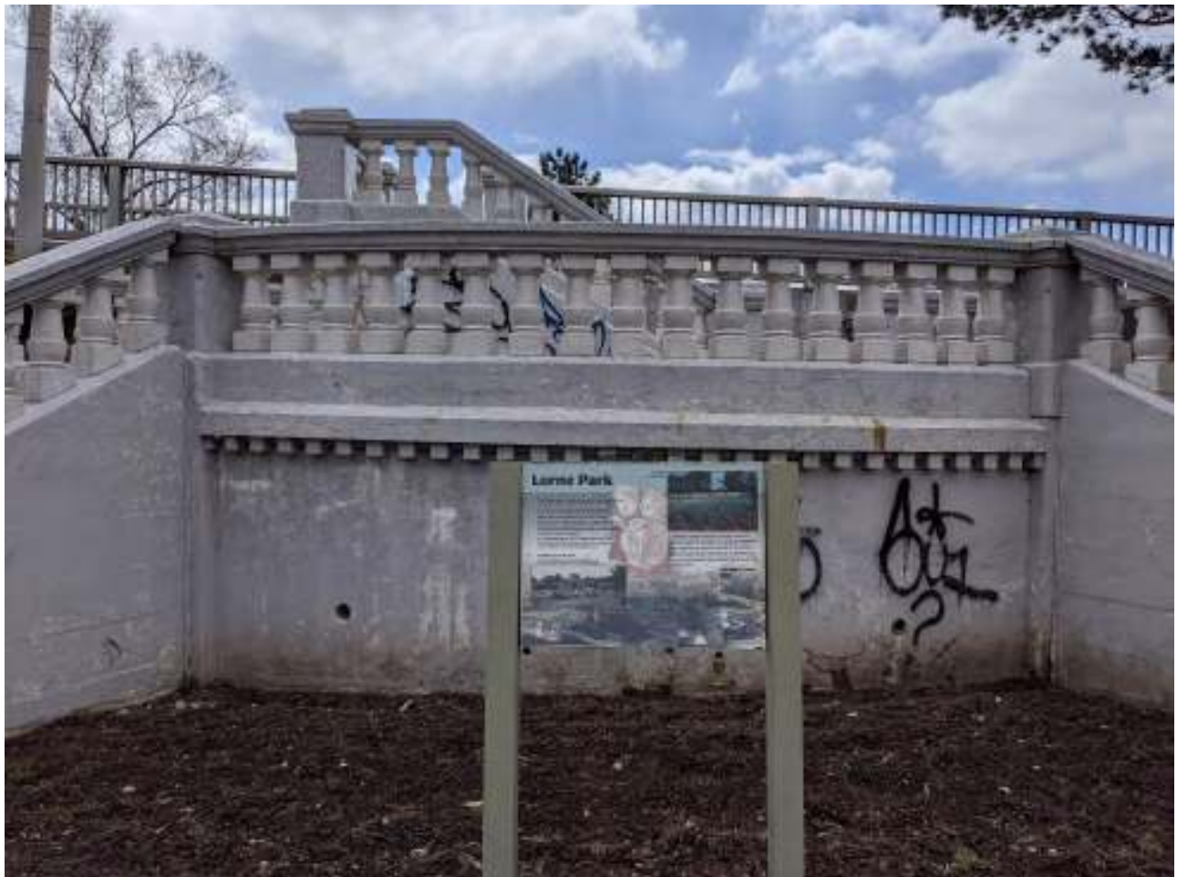
Figure 25: Outer face of the landing with denticulated cornice, thick square newels, and low chamfered and moulded handrail with “Renaissance” balusters
