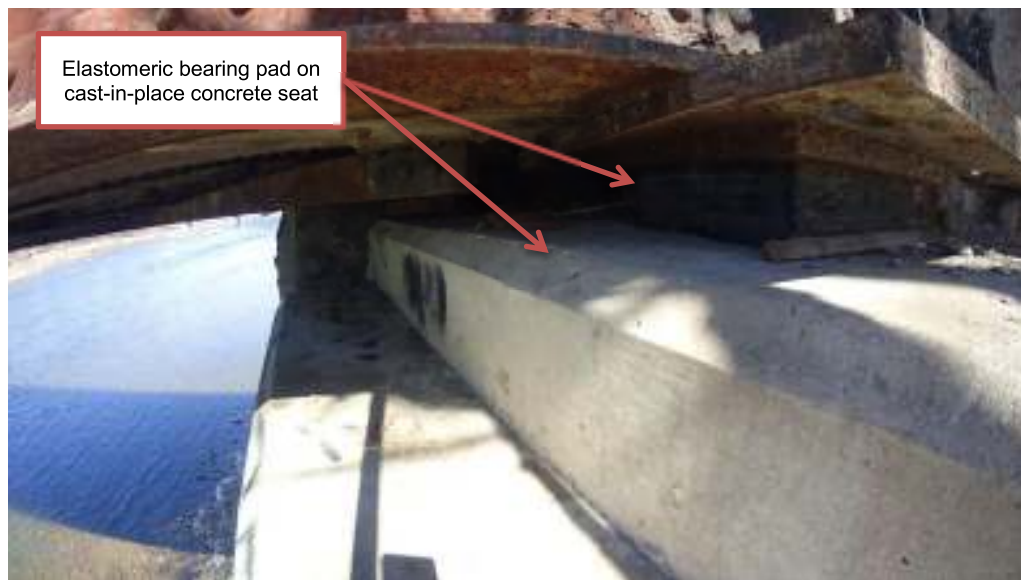
Figure 2: Replaced abutment bearing on Bridge 143
