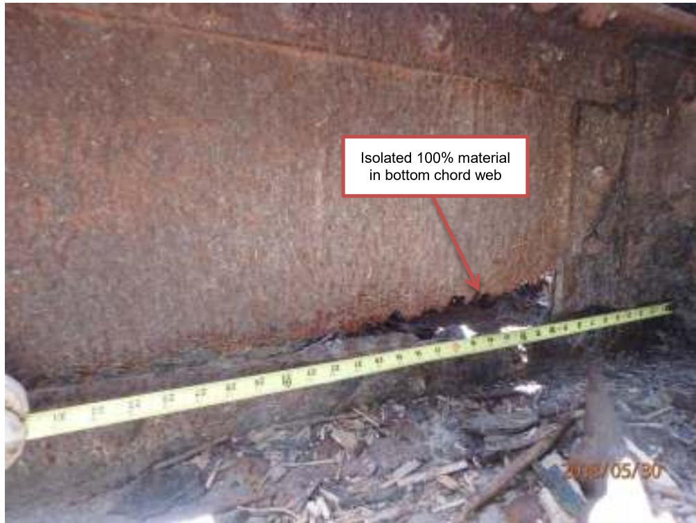
Photograph T9: West truss, bottom chord
