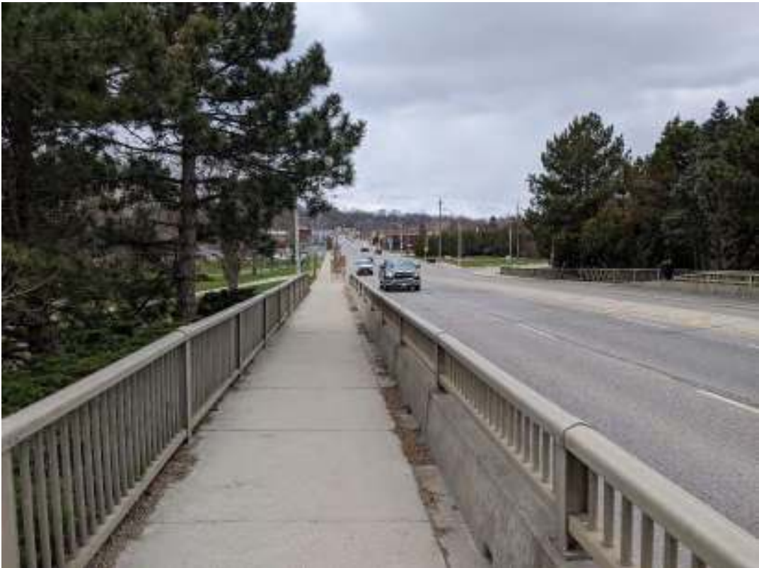
Figure 8: View west from the Lorne Bridge
