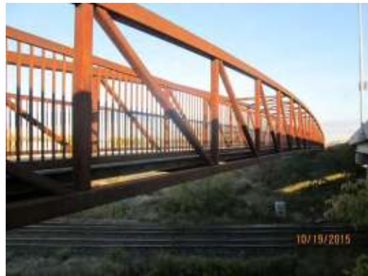
Figure 3: Prefabricated steel truss superstructure (Structure 152)
