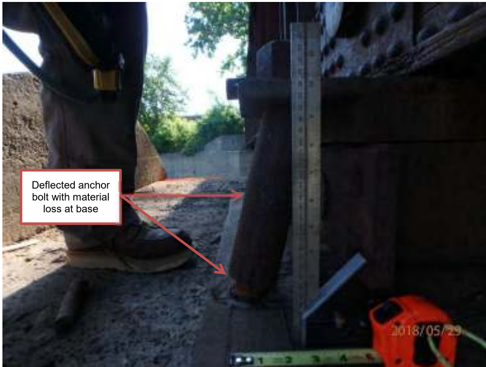
Photograph T3: East pier, north roller bearing
