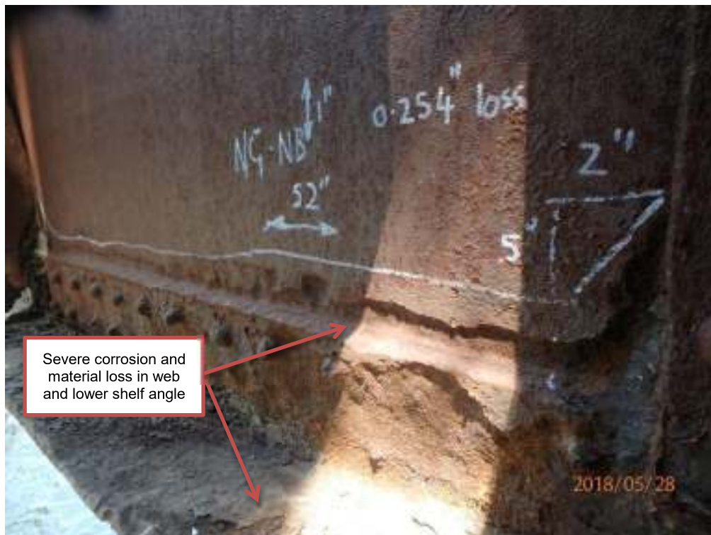
Photograph G8: East span, north girder interior
