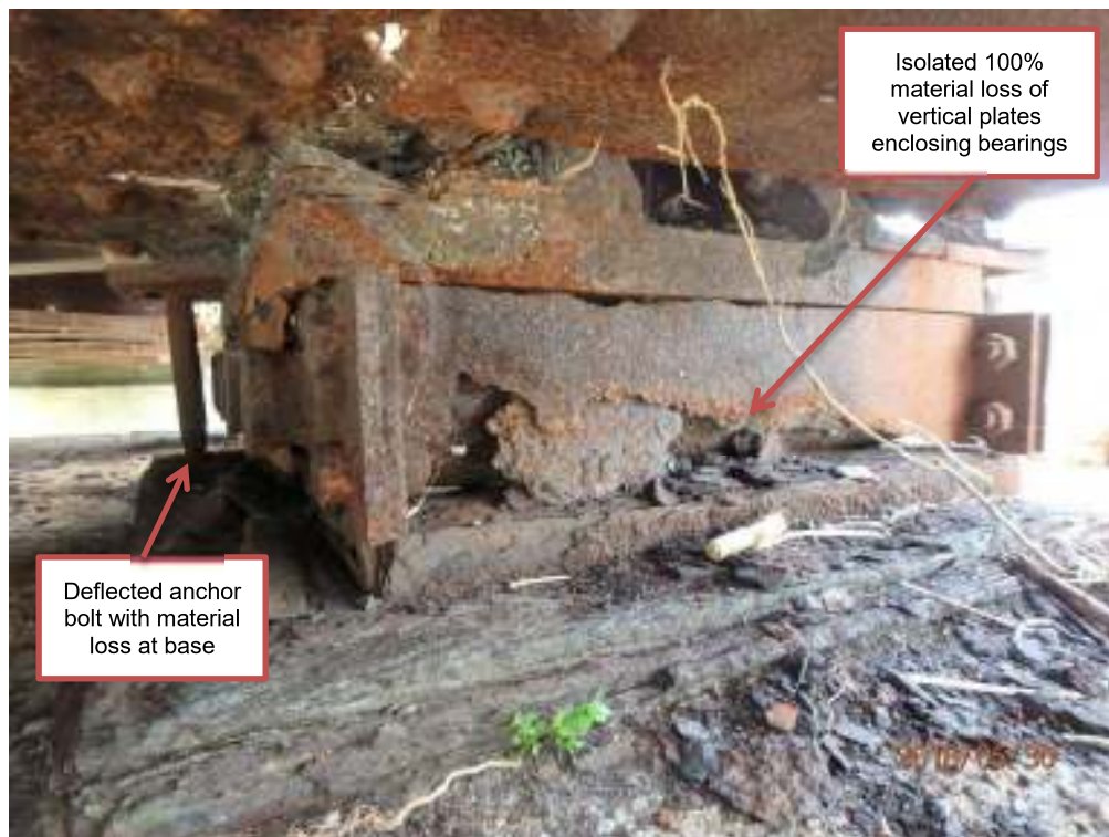
Photograph T4: West pier, north roller bearing
