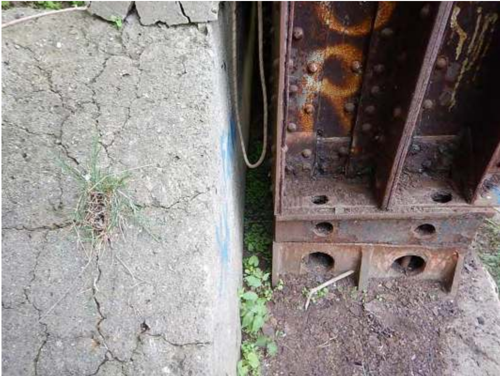
Photograph G5: West abutment, south bearing
