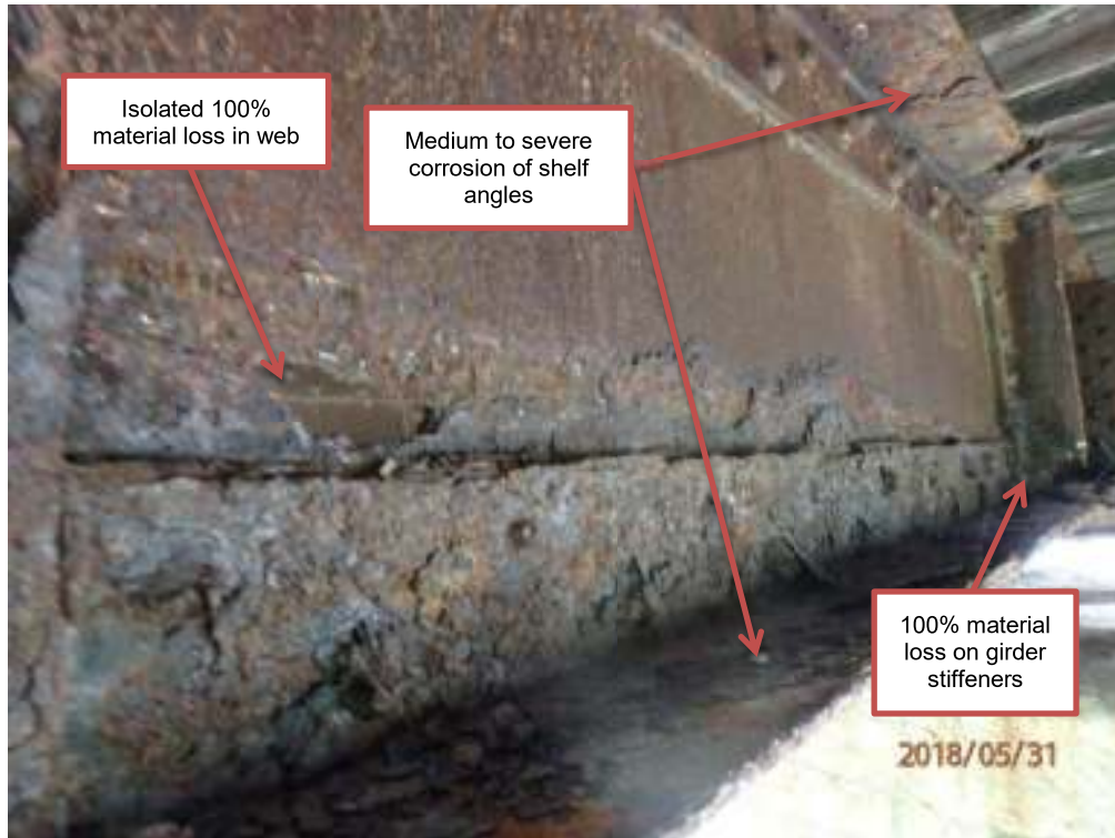
Photograph G11: West span, south stringer
