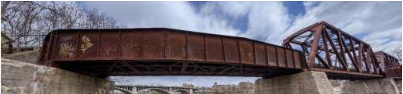
Figure 41: West approach girder span (includes some camera distortion).
