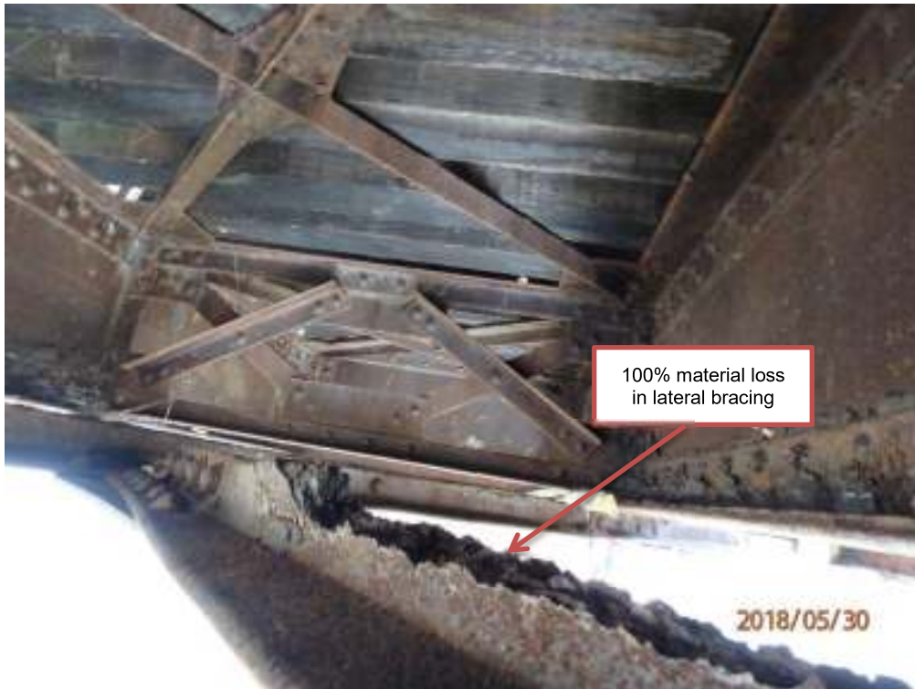
Photograph T13: East truss, lateral bracing
