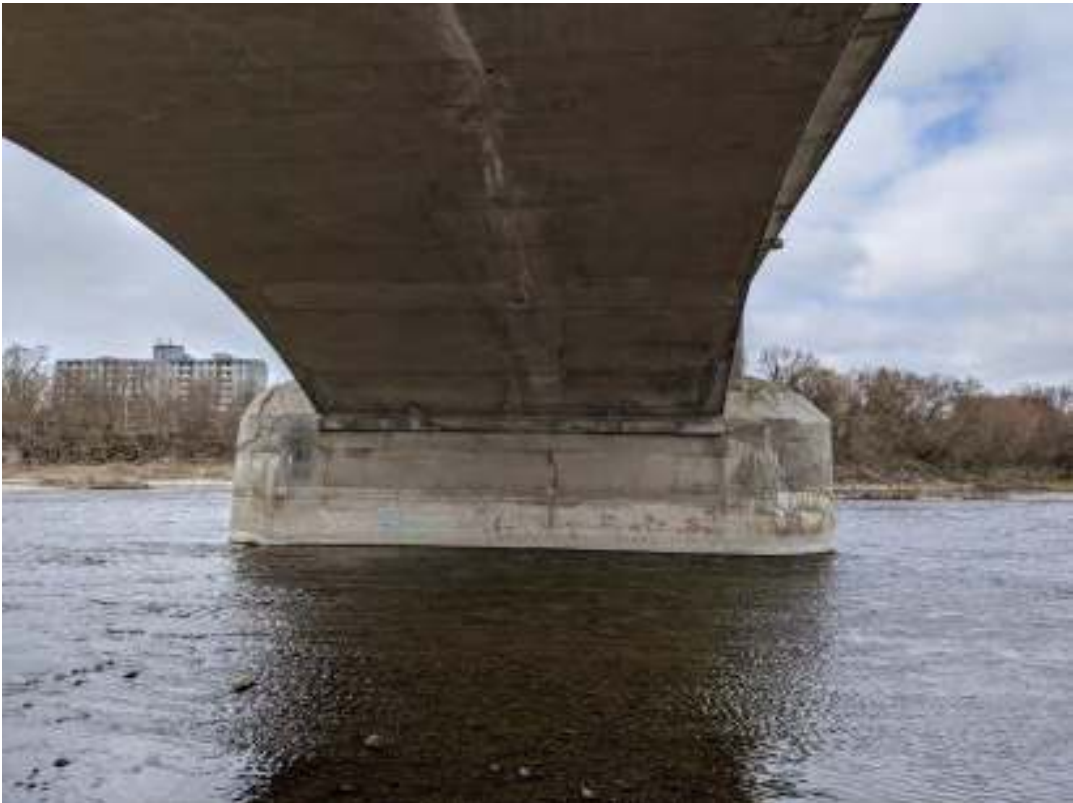
Figure 18: Spring of the arch at Pier No. 1
