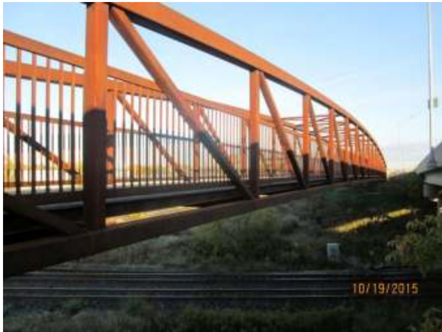
Figure 76: Example of a prefabricated steel through truss pedestrian bridge (courtesy GM BluePlan)
