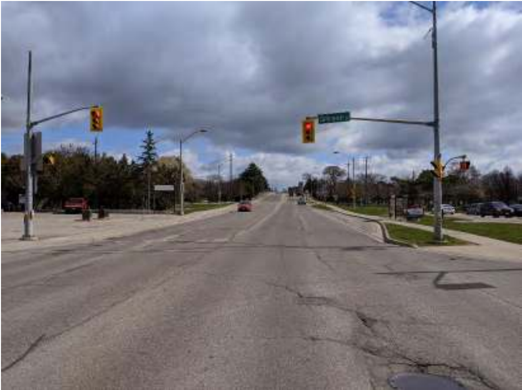
Figure 7: View facing east of the west approach
