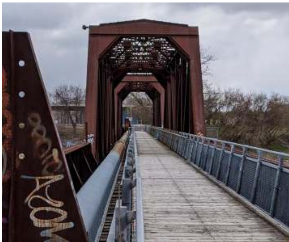
Figure 51: West portal of the west span
