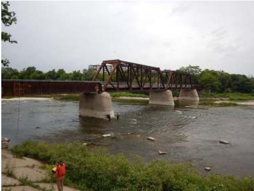
Photograph G1: North elevation
