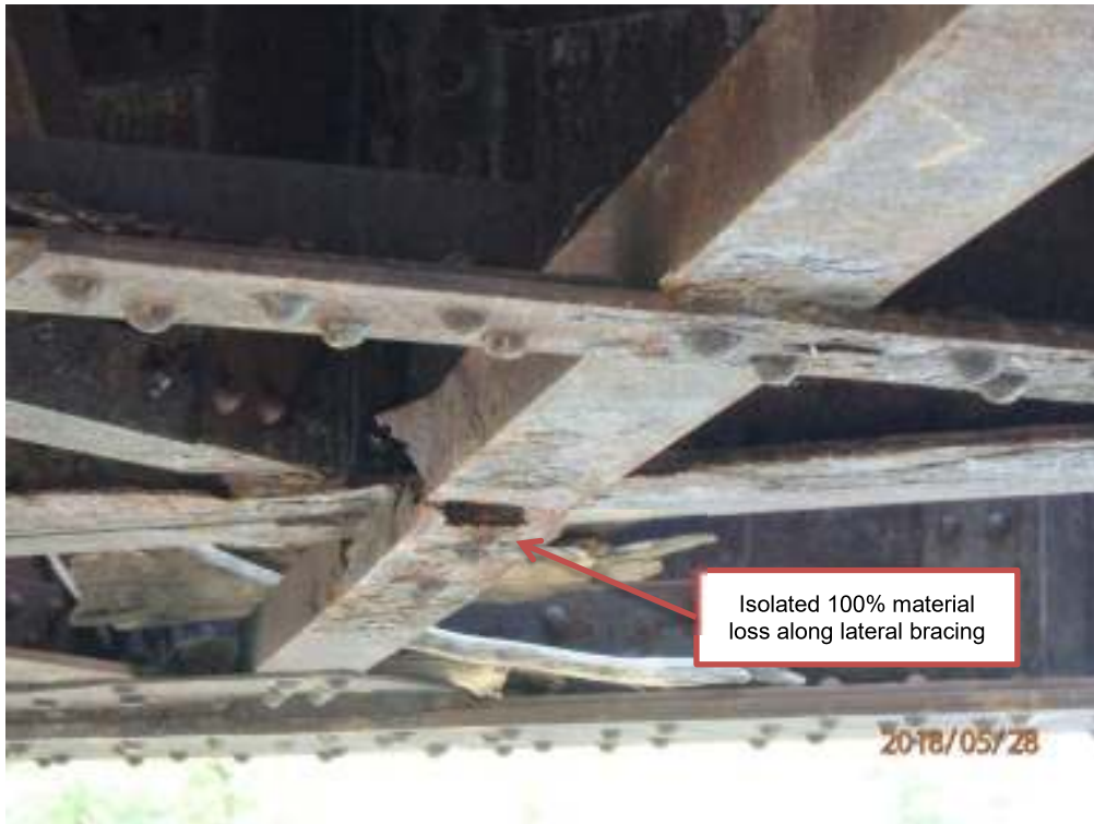
Photograph G13: East span, underside
