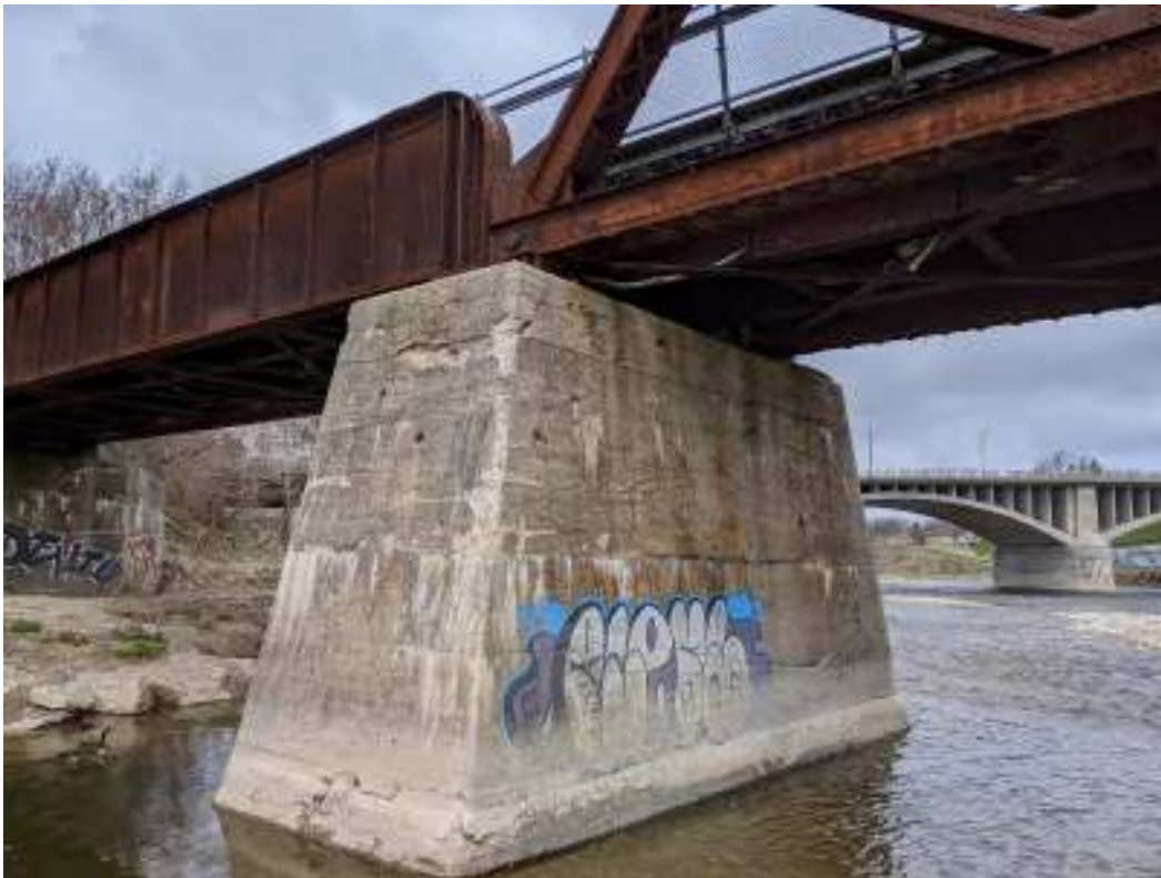
Figure 40: Downriver and east side of Pier No. 3
