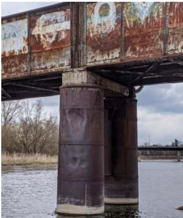
Figure 69: View facing south of the central TH&B Crossing Bridge pier bent caissons
