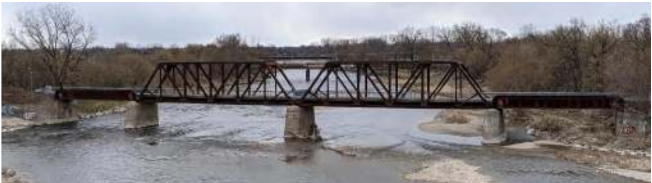
Brant's Crossing Bridge, North Elevation
