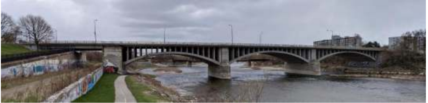
North elevation of the Lorne Bridge
