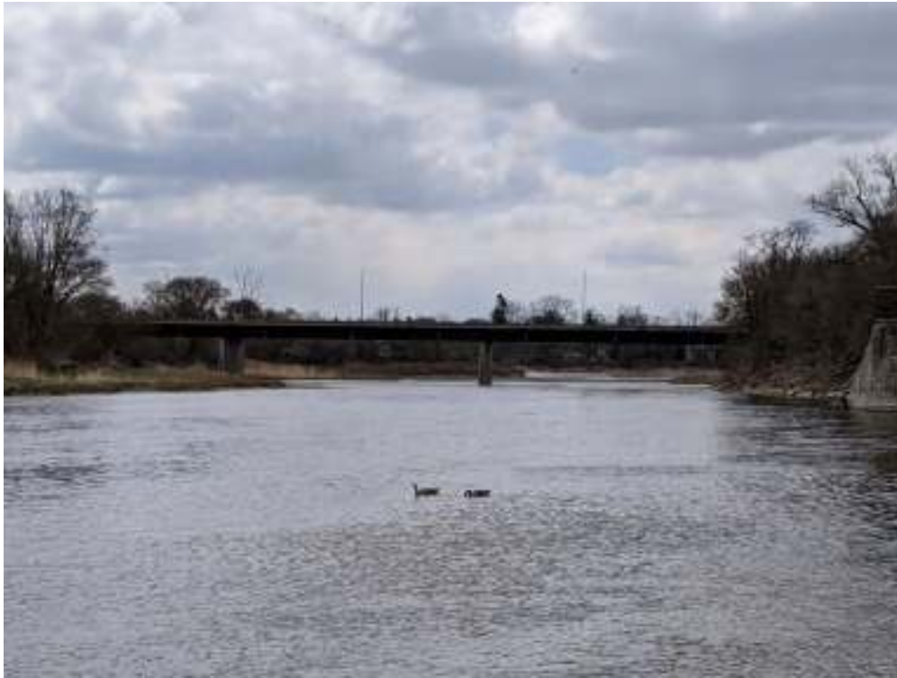
Figure 59: View facing south from the TH&B Crossing Bridge of the BSAR Bridge
