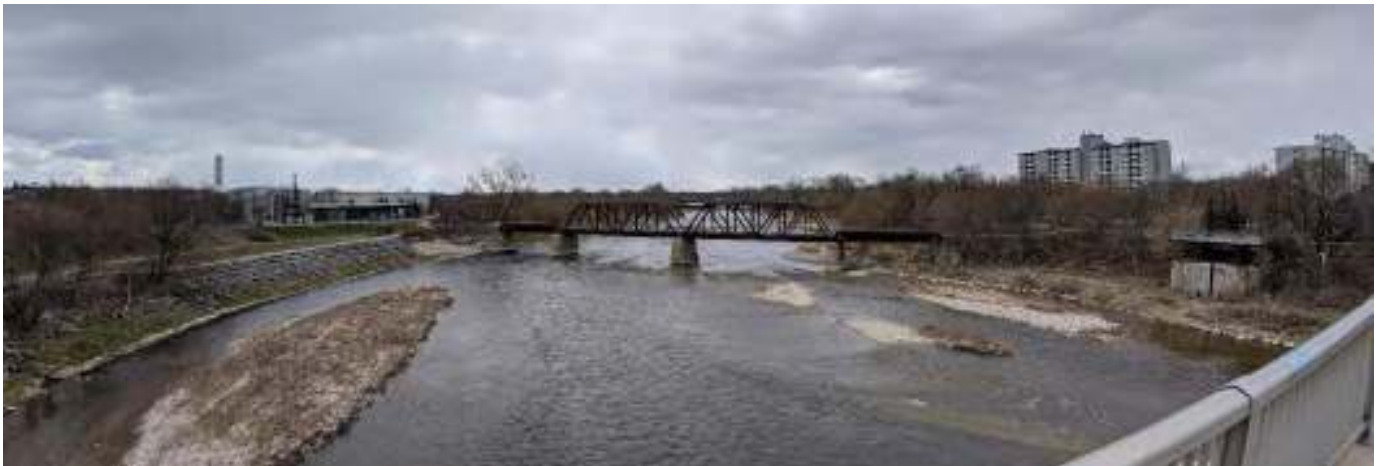
Figure 10: Vista facing south from the Lorne Bridge
