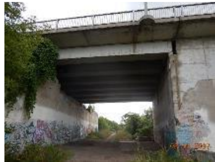
Figure 1-3: Lorne Girder Bridge
