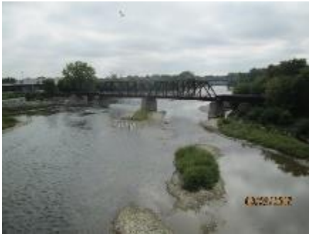
Figure 1-5: Brant's Crossing Bridge, Looking South
