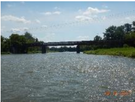
Figure 1-8: TH&B Crossing Bridge, Looking South
