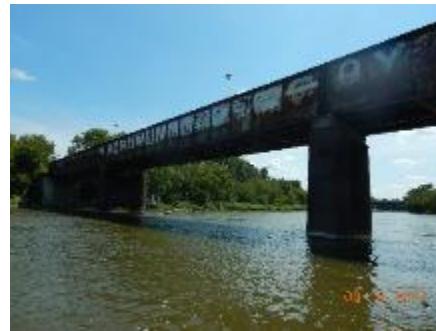
Figure 1-9: TH&B Crossing Bridge, Looking South
