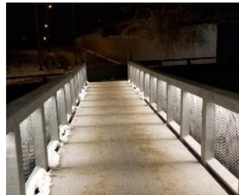
Figure 8-6: Example of Aesthetic Lighting Mounted on a Pedestrian Bridge in Guelph
