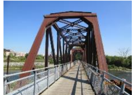
Figure 1-7: Brant's Crossing Bridge, Looking East
