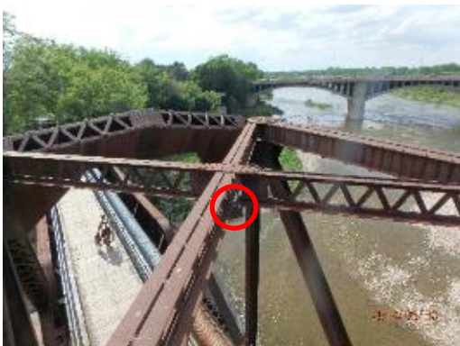
Figure 8-5: Example of Existing Lighting Mounted on Brant's Crossing Bridge
