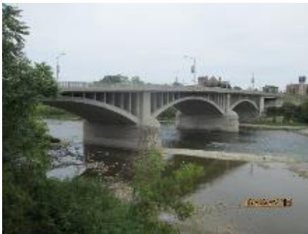
Figure 1-2: Lorne Arch Bridge
