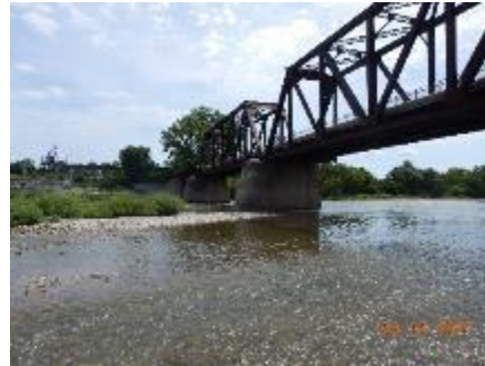
Figure 1-6: Brant's Crossing Bridge, Looking East
