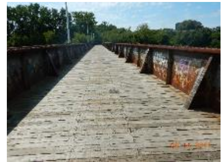
Figure 1-10: TH&B Crossing Bridge, Looking West
