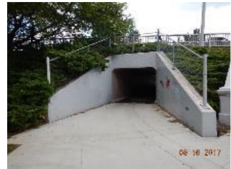
Figure 1-4: Lorne Bridge Pedestrian Underpass
