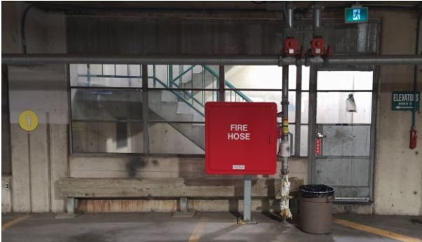
Figure 22 - Market Centre Parkade - Level 1 Yellow Sign & Pedestrian Access
