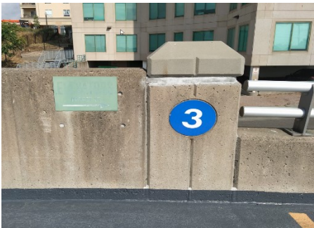
Figure 24 - Market Centre Parkade - Level 3 Blue Sign
