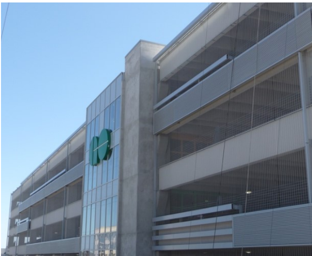
Figure 11 – Ajax GO Station – Precast Concrete Garage
