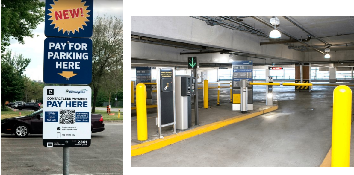
Figure 21 - Examples of Pay By Mobile Phone (Scan QR code) & Automated Pay-on-Foot System
