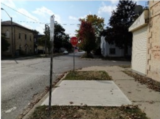
BS718 – Park Ave, SB & Nelson St
