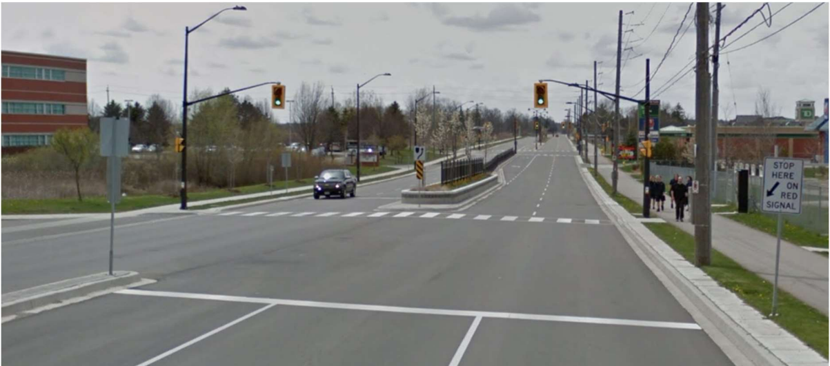
Figure 3-11: Intersection Pedestrian Signal – Shellard Lane at Assumption College Brantford, ON
