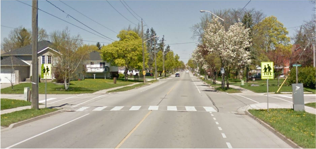
Figure 3-8: Uncontrolled Crossing (with Signage) – Erie Avenue at Dorothy Street Brantford, ON
