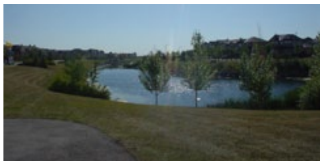
Stormwater management pond as a neighbourhood feature
