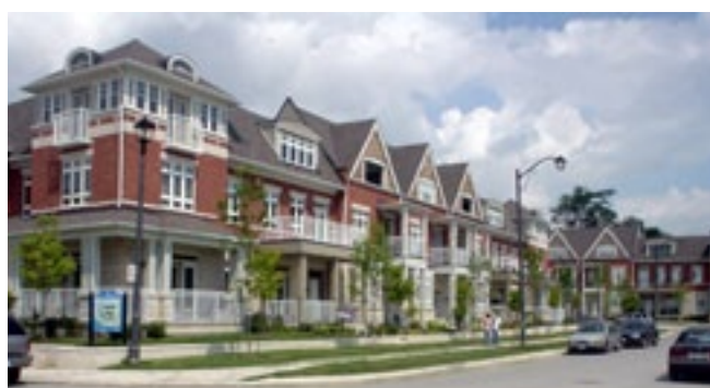
Houses located close to the front property line at a consistent setback, rearlanes provide access to garages
