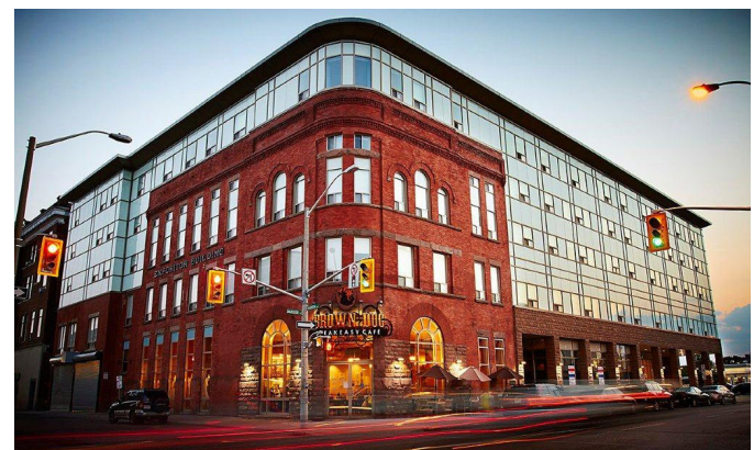
Expositor Place Building
