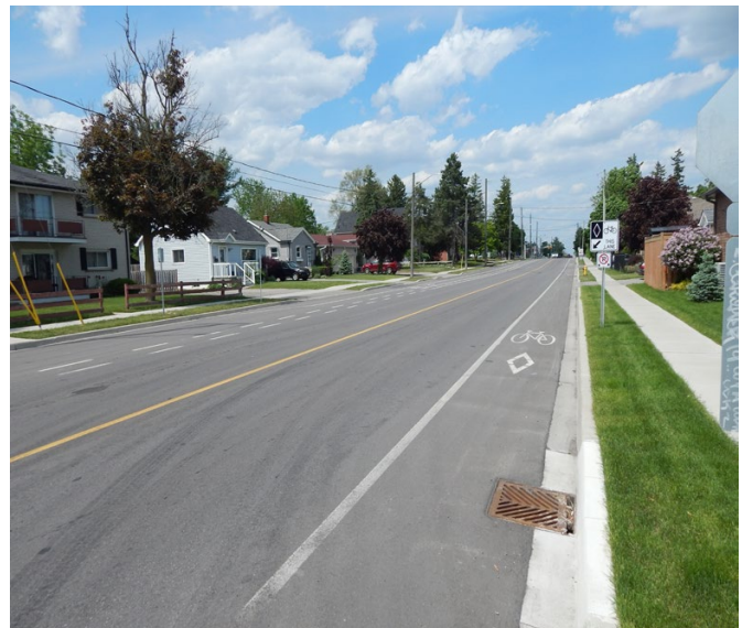
Accessible sidewalks should be provided on both sides of the street with adequate boulevard separation / Brantford, ON.
