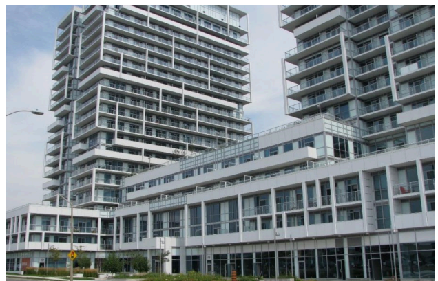
A variety of design approaches can be applied to the podium and tower portions of buildings such as stepbacks, setbacks, separation distances and differing placement and orientation
