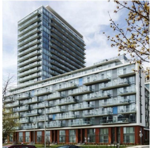
Buildings should include well designed and articulated podiums, middle sections, and tops
