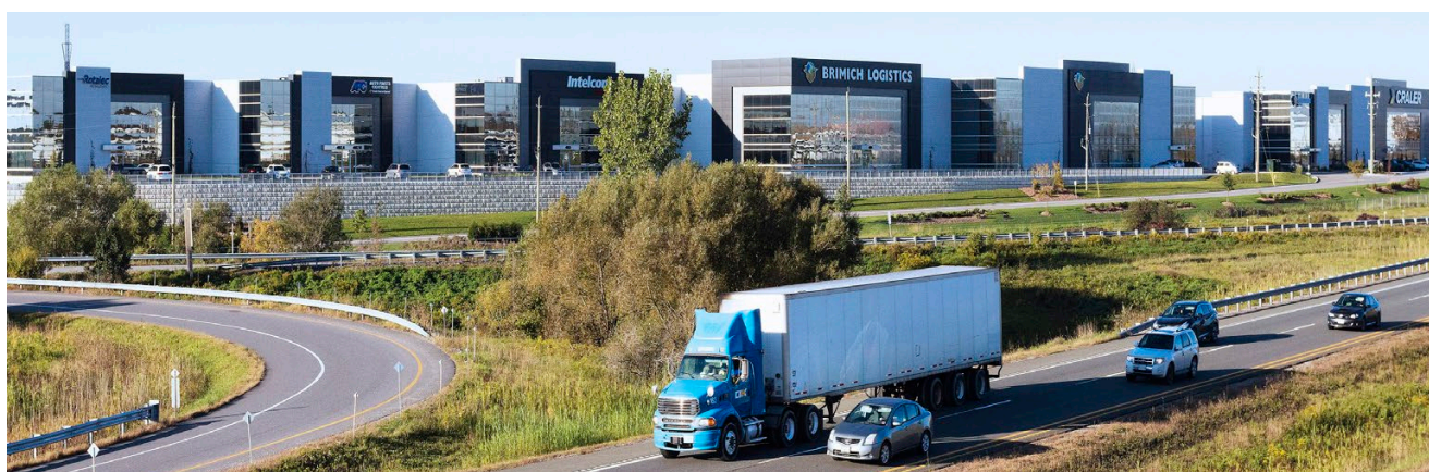
Employment buildings with publicly visible façades should be articulated through high quality design
