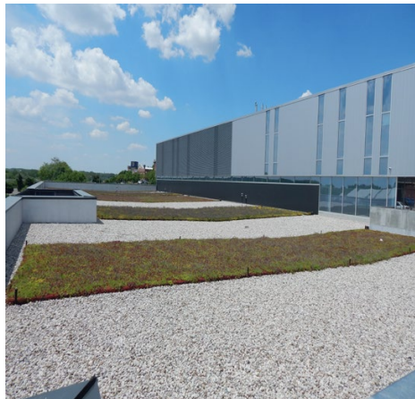
Laurier Brantford YMCA Green Roof
