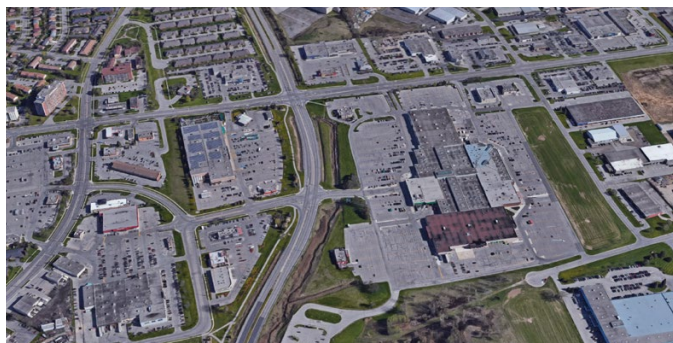
Lynden Park Mall and surrounding area
