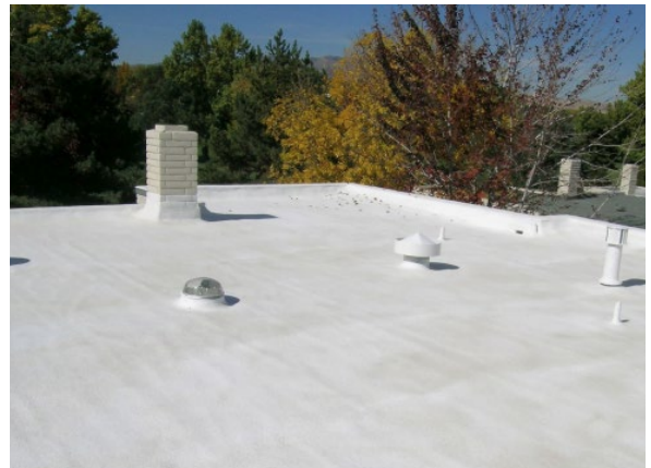
Light coloured roofs have a high solar reflectance, which reduces energy costs and the urban heat island effect.
