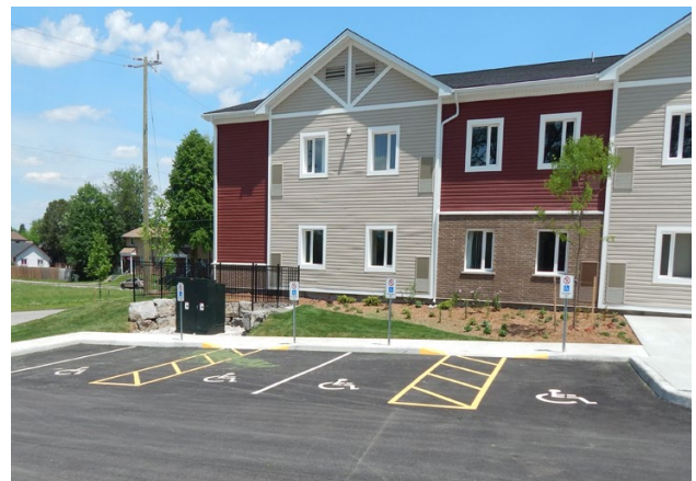
Accessible parking should be provided in proximity to an accessible and sloped building entrance
