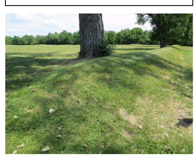
Berm to manage and redirect overland flows. Could be used at the top of slope to minimize runoff onto the slope.
