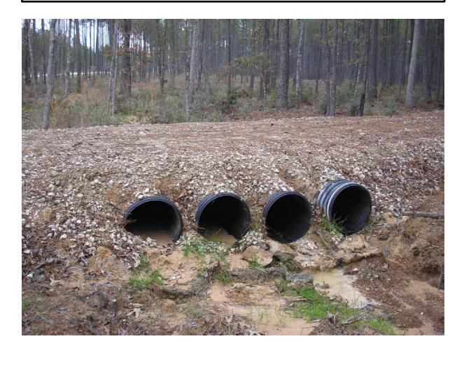
Culverts installed at locations along the trail to drain pooled water along the trail. Would reduce soil moisture on the slope.
