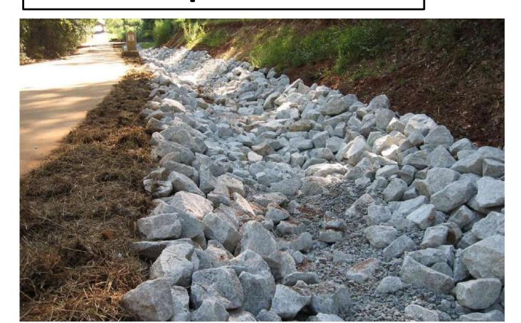
Interceptor Trench to collect and drain near-surface water at the top of slope and at the trail.
