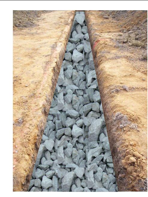
Series of rock drainage features on the lower slope to reduce soil moisture. Would be required to support mechanical stabilization.
