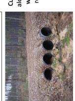
Culverts installed at locations along the trail to drain pooled water along the trail. Would reduce soil moisture on the slope.
