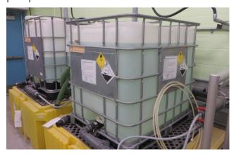
For chemicals that have the potential to release gases, provide air scrubbers for chemical storage areas to suit the type and size of the chemical stored and in accordance with the Ontario Design Guidelines for Drinking Water Systems and the Ontario Design Guidelines for Sewage Works.
