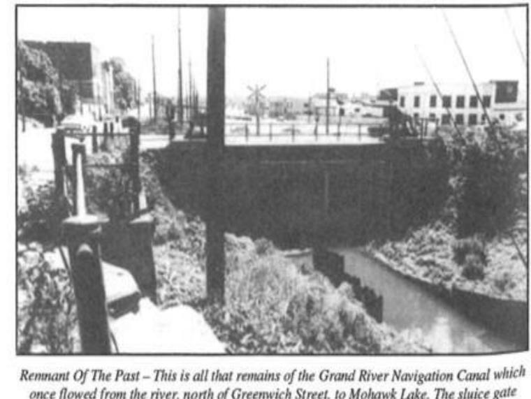
once flowed from the river, north of Greenwich Street, to Mohawk Lake. The sluice gate allows water to run through a buried pipeline to Mohawk Lake, whenever the river rises.
