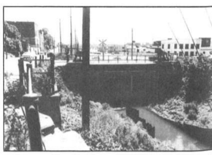
Remnant Of The Past – This is all that remains of the Grand River Navigation Canal which once flowed from the river, north of Greenwich Street, to Mohawk Lake. The sluice gate allows water to run through a buried pipeline to Mohawk Lake, whenever the river rises.
