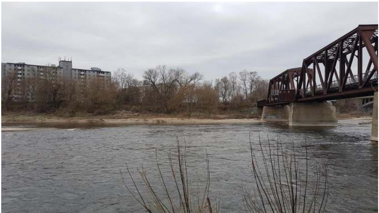
Image 8: A representative example of the City of Brantford's dike system; facing west, April 24, 2020.
