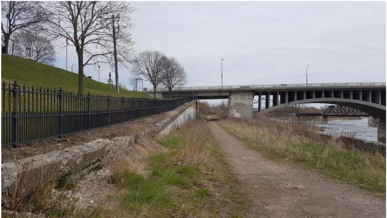
Image 13: The former Lake Erie and Northern Railway converted to a recreational path within the Study Area; facing southeast, April 24, 2020.
