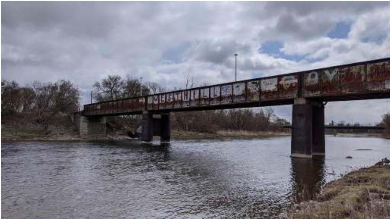
Image 11: The TH&B Crossing Bridge; facing southeast, April 24, 2020.
