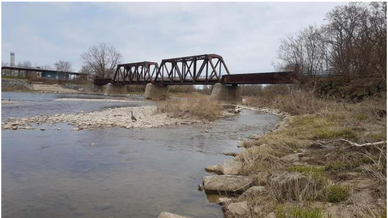
Image 10: The Brant's Crossing Bridge; facing east, April 24, 2020.
