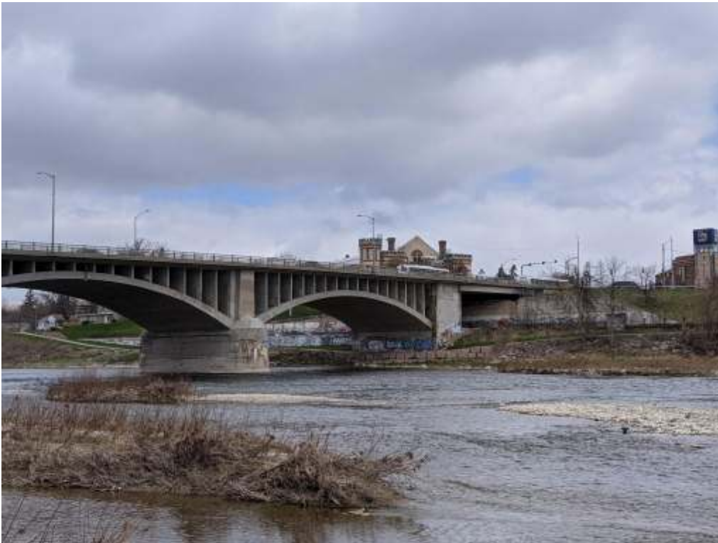
Photograph 8: Lorne bridge - Looking towards east pier and abutment from downstream side.
