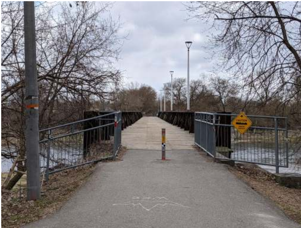
Photograph 17: TH&B Crossing Bridge – Looking west.
