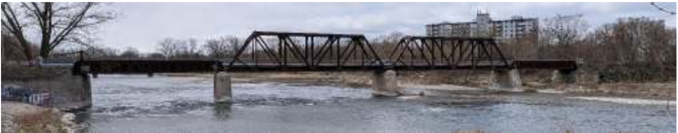
Photograph 2: View from the former railbed of the LE&N atop the stone embankment to the northeast of the bridge, facing southwest.
