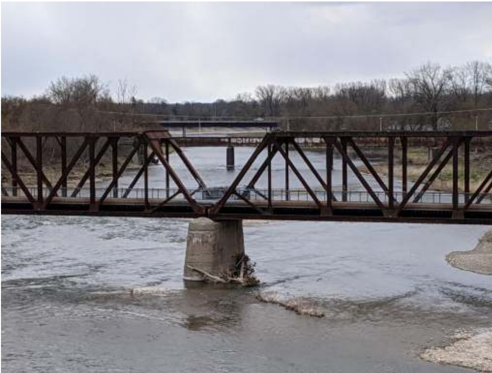
Photograph 12: Brant's bridge – Looking at central pier looking from upstream side.
