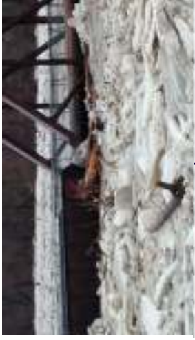
Deflection of Anchor Bolt
