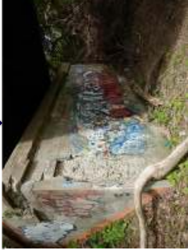
Deterioration of Concrete Abutment
