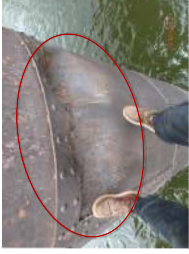
Deterioration of Concrete Abutment
