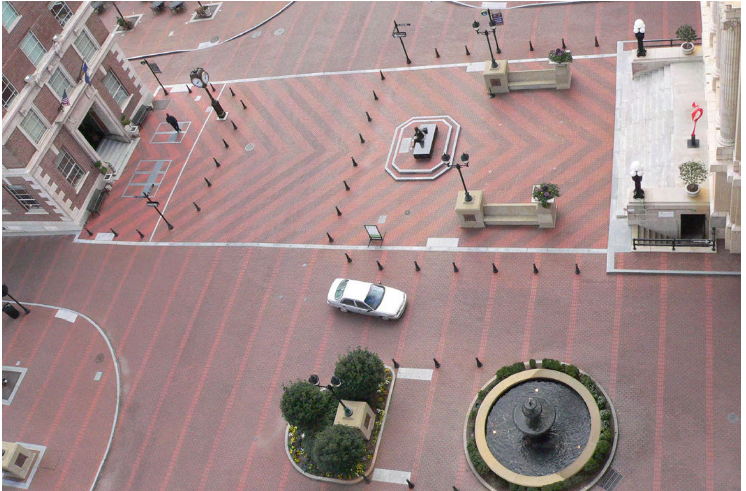
Paving design can be used to enhance the visual experience within the public realm and also delineate special areas and functions within the downtown.
