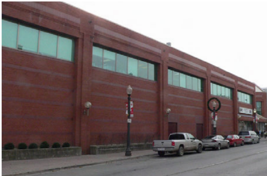
Changing past practices: existing ground condition with poor street relationship. Downtown Brantford.
