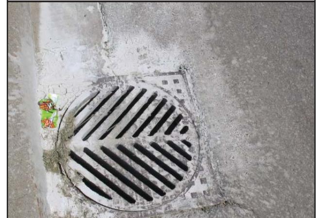
Discharge of concrete wash water into catch basin. Due to the high pH in concrete wash water, this can have an impact on aquatic life in receiving streams.
