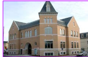
LAURIER STUDENT UNION BUILDING 103 Darling Street
