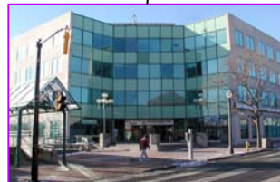
GRAND RIVER HALL 171 Colborne Street (150 residence spaces & teaching facilities)
