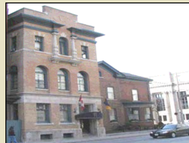
The Hamilton Club Façade Improvement and Renovation
