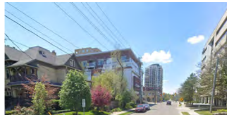
Waterloo - 21 Allen St (6 storey residential building)
