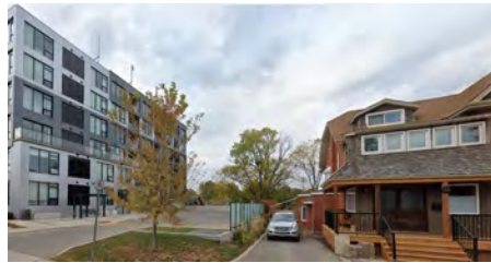
Kitchener - 12 Lousia St (6 storey Residential building)
