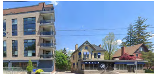
Kitchener - 217 King St S (6 storey Mixed Use Building)
