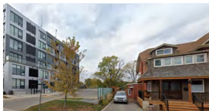
Kitchener - 12 Lousia St (6 storey Residential building)
