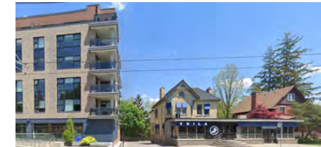
Kitchener - 217 King St S (6 storey Mixed- use Building)
