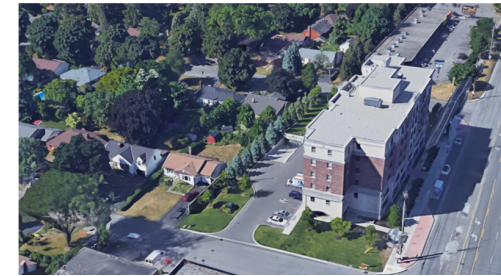
Burlington - Kingsway Dr and Plains Rd East (6 Storey Mixed use building)
