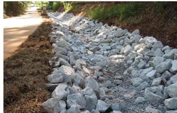
Interceptor Trench to collect and drain near-surface water at the top of slope and at the trail.
