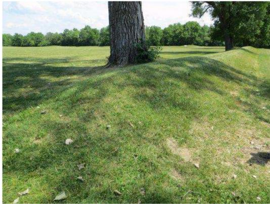
Berm to manage and redirect overland flows. Could be used at the top of slope to minimize runoff onto the slope.
