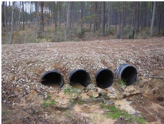
Culverts installed at locations along the trail to drain pooled water along the trail. Would reduce soil moisture on the slope.
