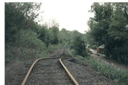
Railway along Beach Road after 1986 landslide
