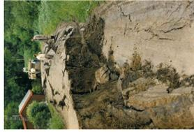
Major slope failure on South side of Colborne Street. Initiates investigations into slope failure within study area. Slope monitoring begins with installation of monitoring equipment.
