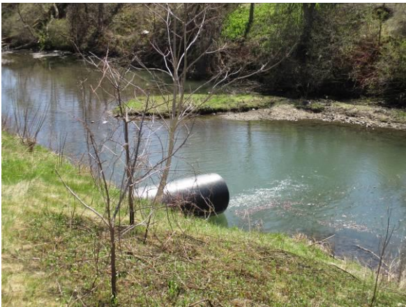
Plate 12: Storm Water Management Outlet (ASI 2016)
