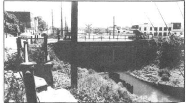
*Remnant Of The Past – This is all that remains of the Grand River Navigation Canal which once flowed from the river, north of Greenwich Street, to Mohawk Lake. The sluice gate allows water to run through a buried pipeline to Mohawk Lake, whenever the river rises.*
