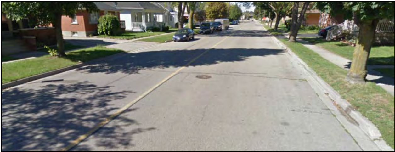
Figure 12. Good Condition (PCI between 60 and 79)
