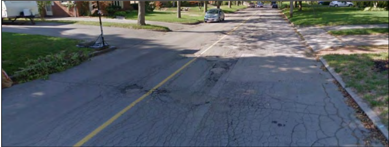
Figure 14. Poor Condition (PCI between 20 and 39)
