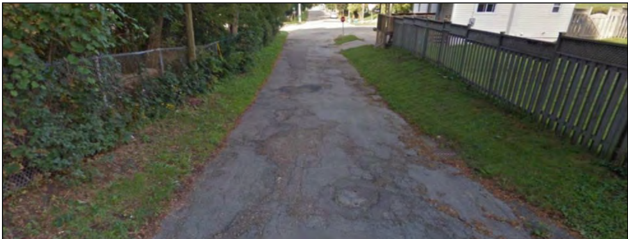
Figure 15. Very Poor Condition (PCI between 0 and 19)
