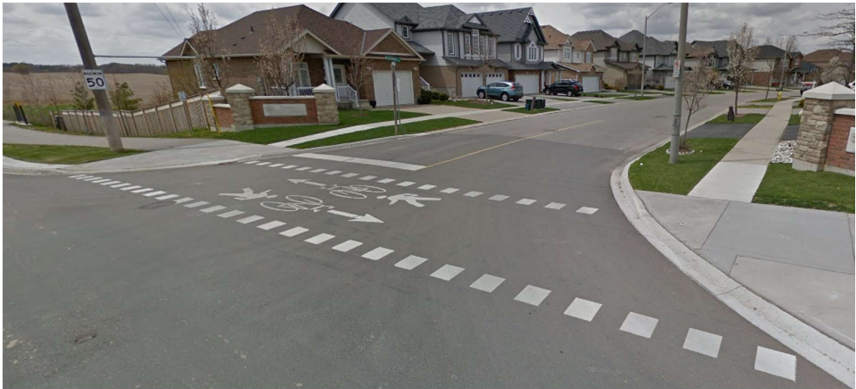
Figure 3-22: Mixed Crossride – Shellard Lane at McGuinness Drive (west) Brantford, ON
