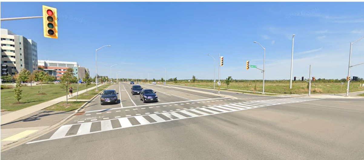
Figure 3-20: Separate Crossride – Dundas Street West at Third Line in Oakville, ON
