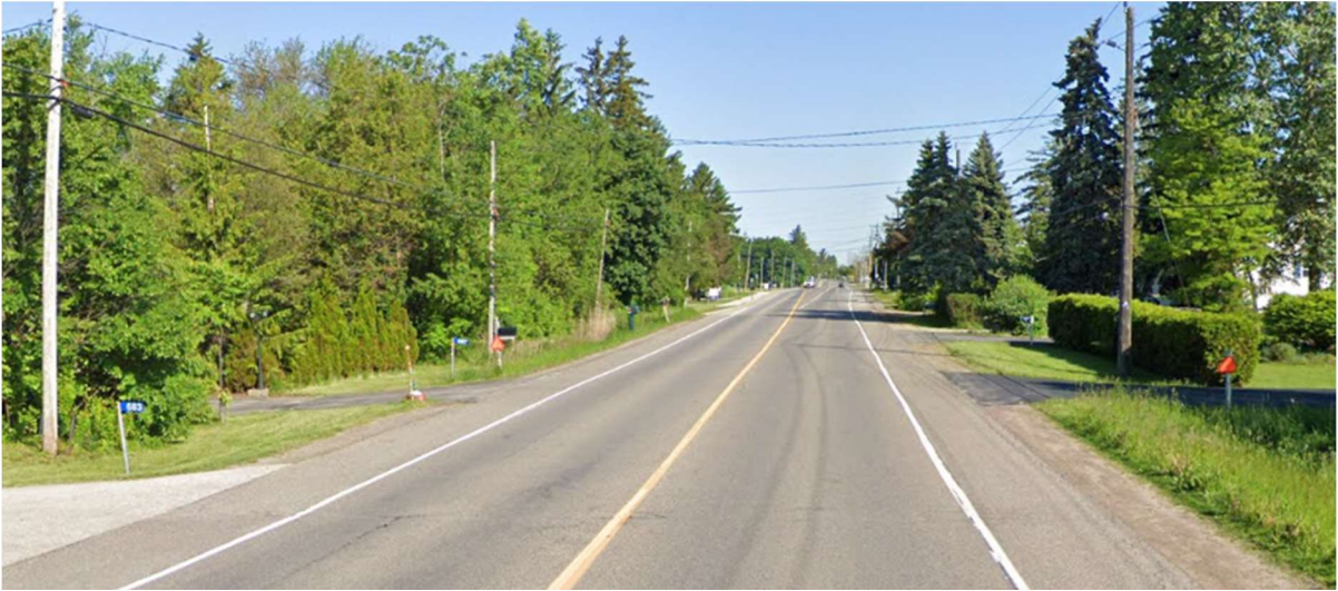
Figure 3-14: Paved Shoulders – Centre Road Waterdown, ON
