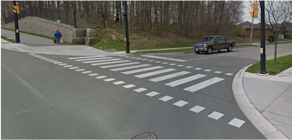
Figure 3-21: Combined Crossride – Shellard Lane at McGuinness Drive (east) Brantford, ON
