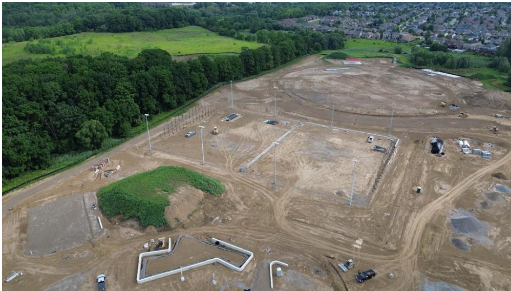
Figure 5 - Blanche E. Williams Community Park Construction Progress Aerial Image
