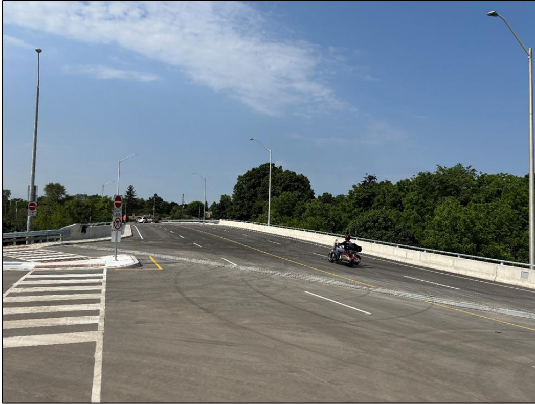
Figure 3 - Ava Road Bridge looking northbound from Brant Avenue
