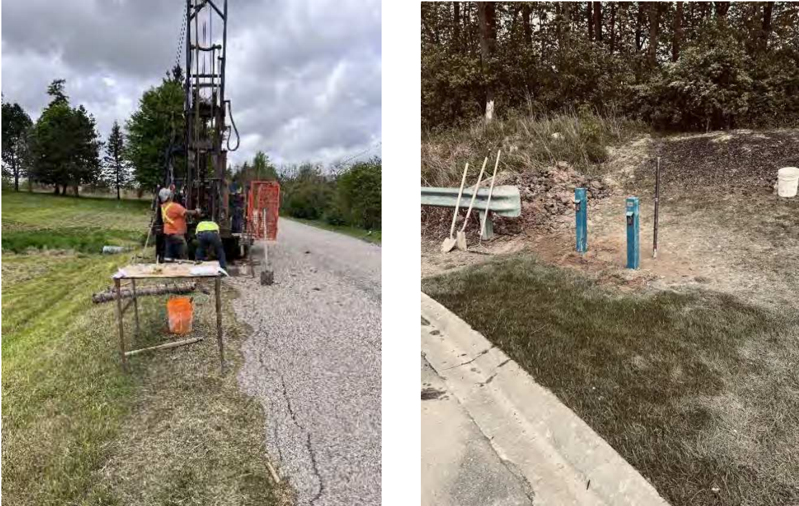
Figure 3.12: Well drilling at MW-1 (left) and well completion at MW-4 (right).
