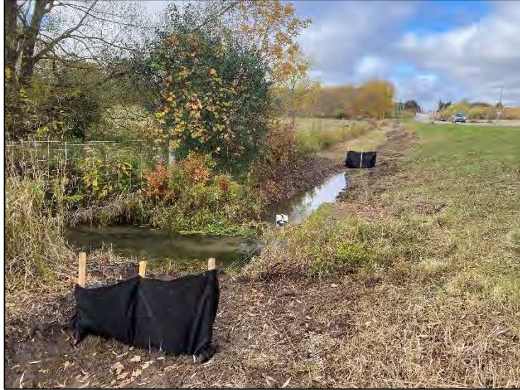
Figure 3.104: Ditching and Sediment Fencing Adjacent to Watercourse
